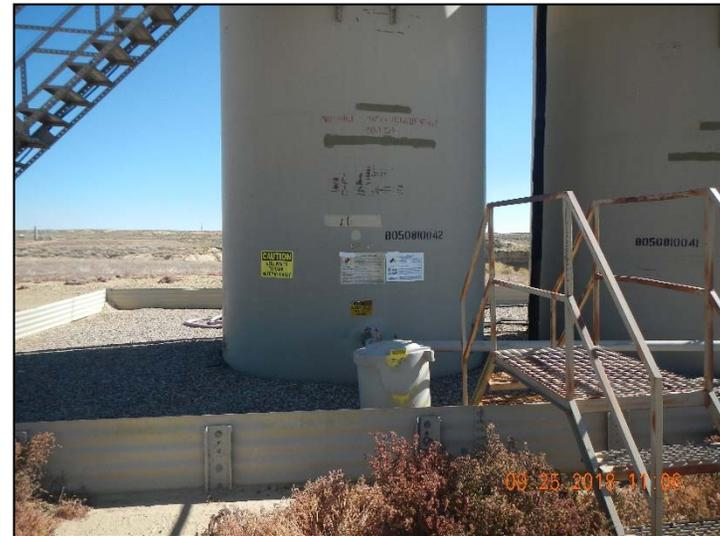
**Photo 2. Tank labeled with two different contents and no capacity; dried annual weeds immediately adjacent to berm.**
