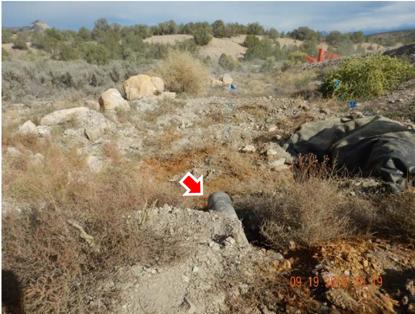
Photo #9 – Additional produced water impacts located ~130' SE of tank battery at distal end of severed 10" poly line (Spill/Release ID #457570). Note operator constructed berm of black liner material to prevent release from entering into stormwater culvert.
