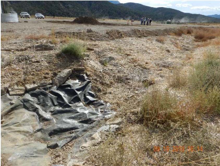
Photo #7 – Dam constructed by operator during initial response to release from severed 10" poly line is located at terminus of stormwater ditch.
