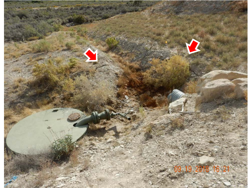
Photo #12 – Subsidence inside of stormwater ditch related to Spill/Release ID #457570.
