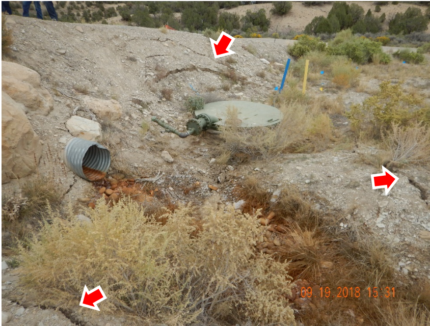
Photo #11 – Valve access vault on south side of lease road was impacted by produced water released during Spill/Release ID #457570. Note evidence of additional subsidence in this area.
