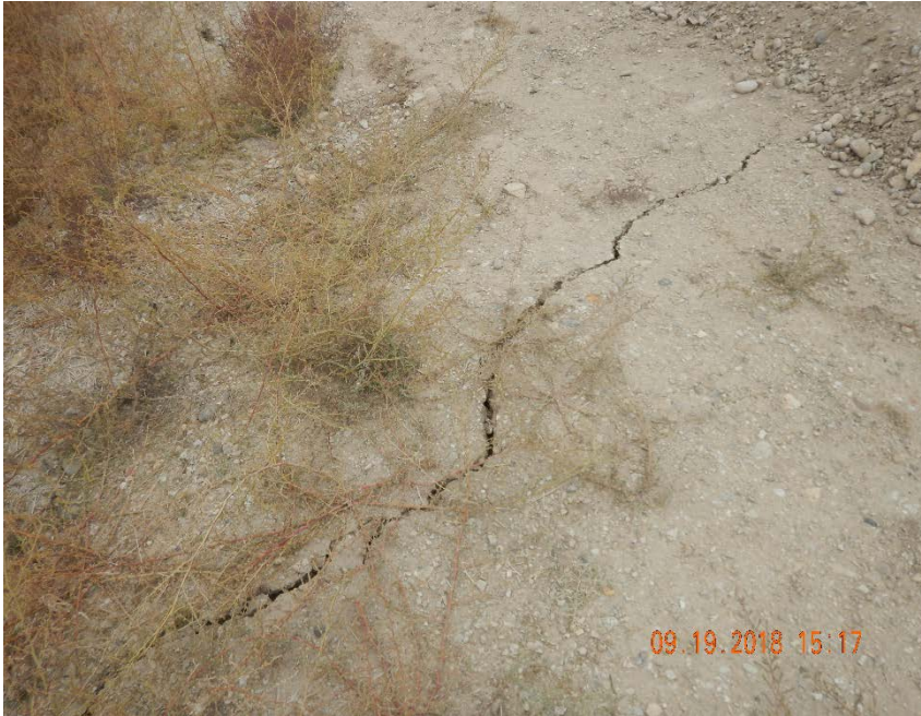
Photo #5 – Subsidence observed along stormwater ditch/former pit area related to subsurface fluid migration. (1)
