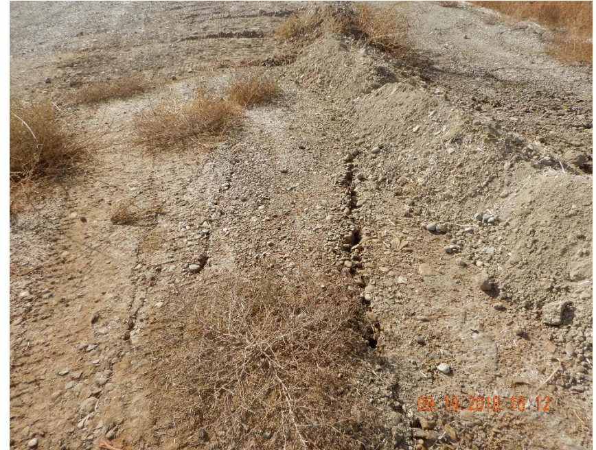
Photo #6 - Subsidence observed along stormwater ditch/former pit area related to subsurface fluid migration. (2)
