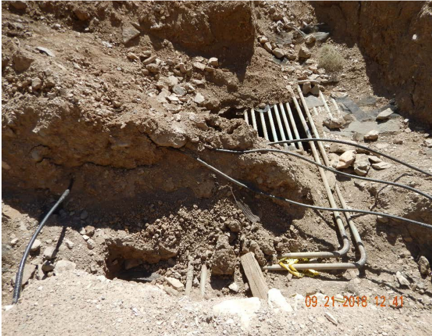
Photo #17 – Looking into open flowline excavation from north side. Note 2" flowlines and black electrical conduit inside of excavation.
