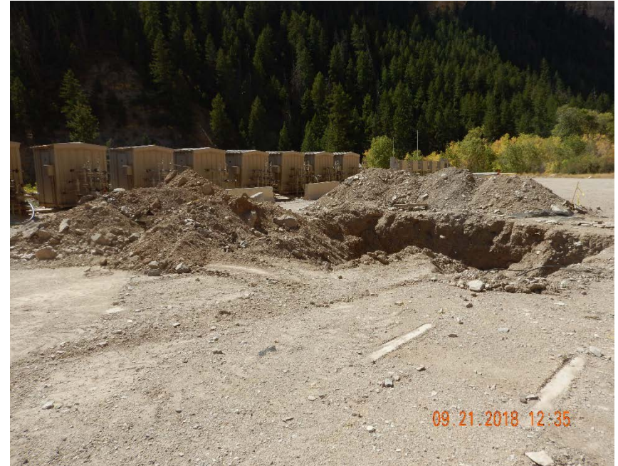
Photo #16 – View of soil stockpiles and open flowline excavation from NE. There was no visible liner beneath either soil stockpile on date of inspection.
