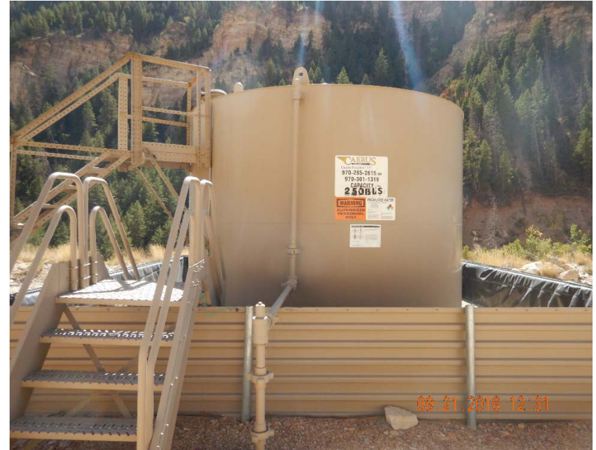
Photo #14 – 250 bbl produced water AST with lined, metal berm.
