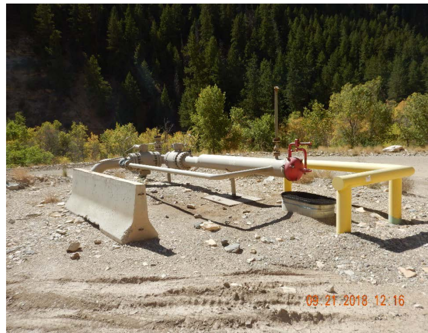
Photo #2 – Pig station located at entrance to pad.
