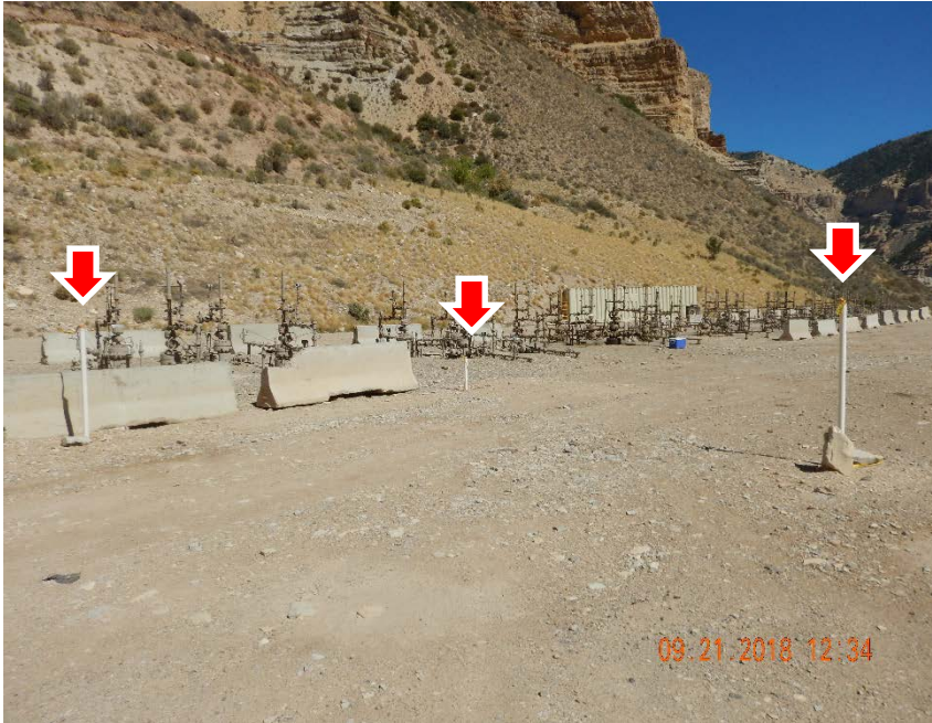
Photo #15 – 2” and 1” PVC risers located in center of pad appear to be temporary monitoring wells.
