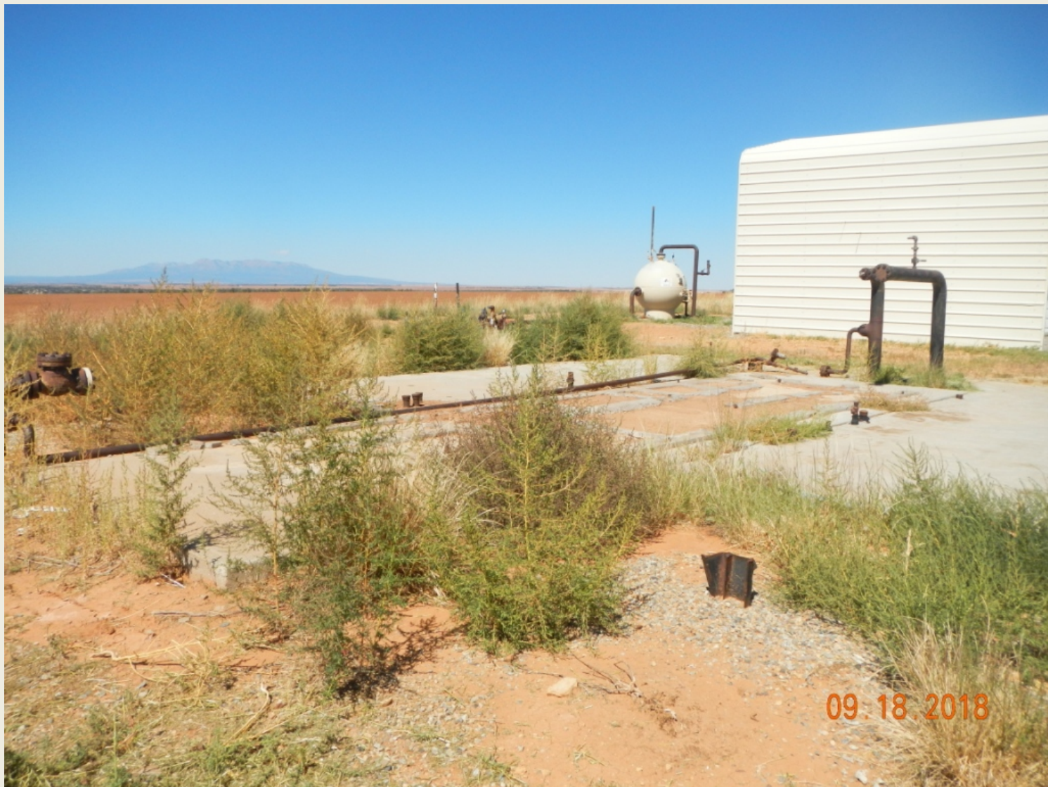
Photo 7. View of what appears to be old tank battery location still in place. Risers and gas lines still in place need proper abandonment.
