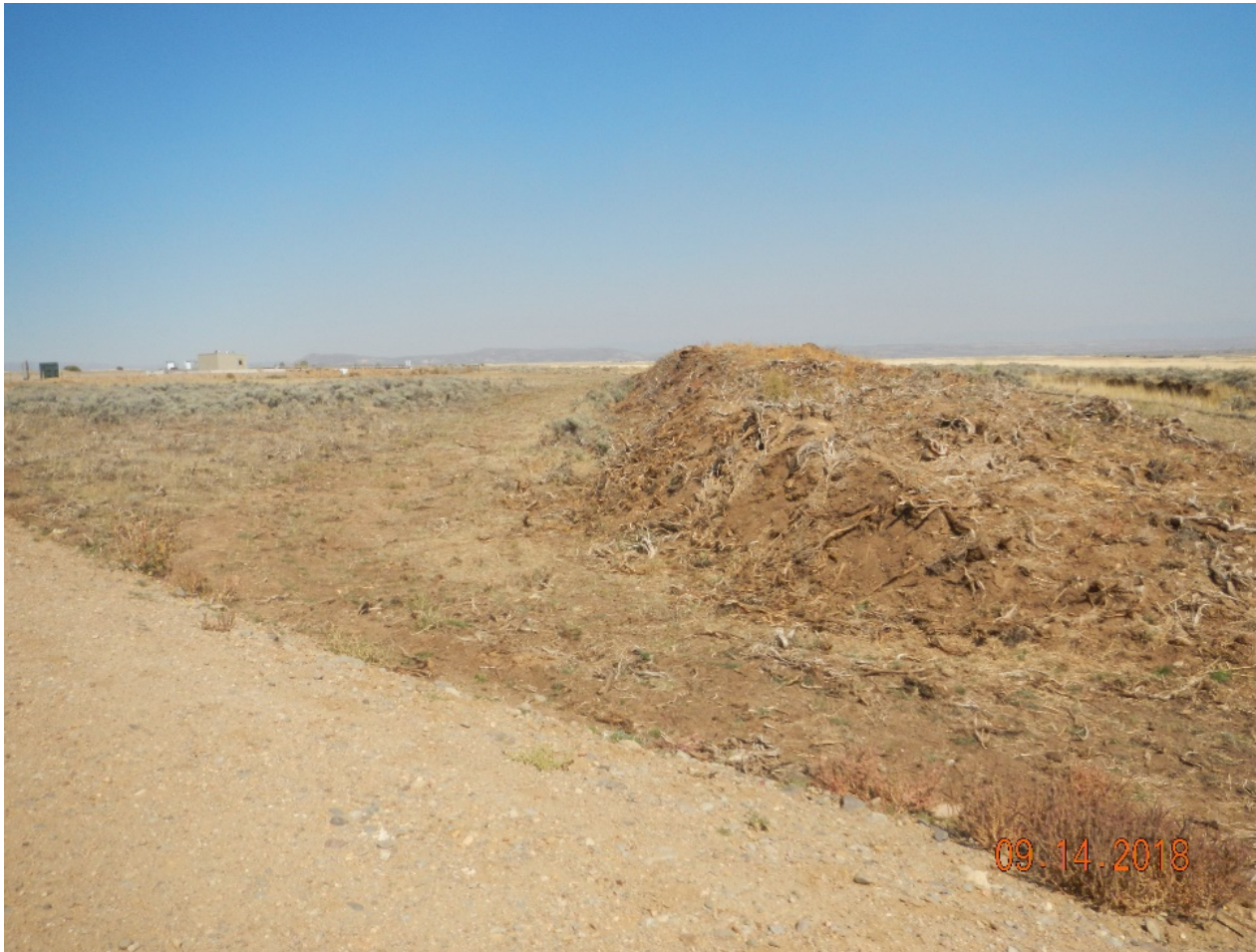
Photo#7: Topsoil pile at South portion of site needs further stabilization & protection.
