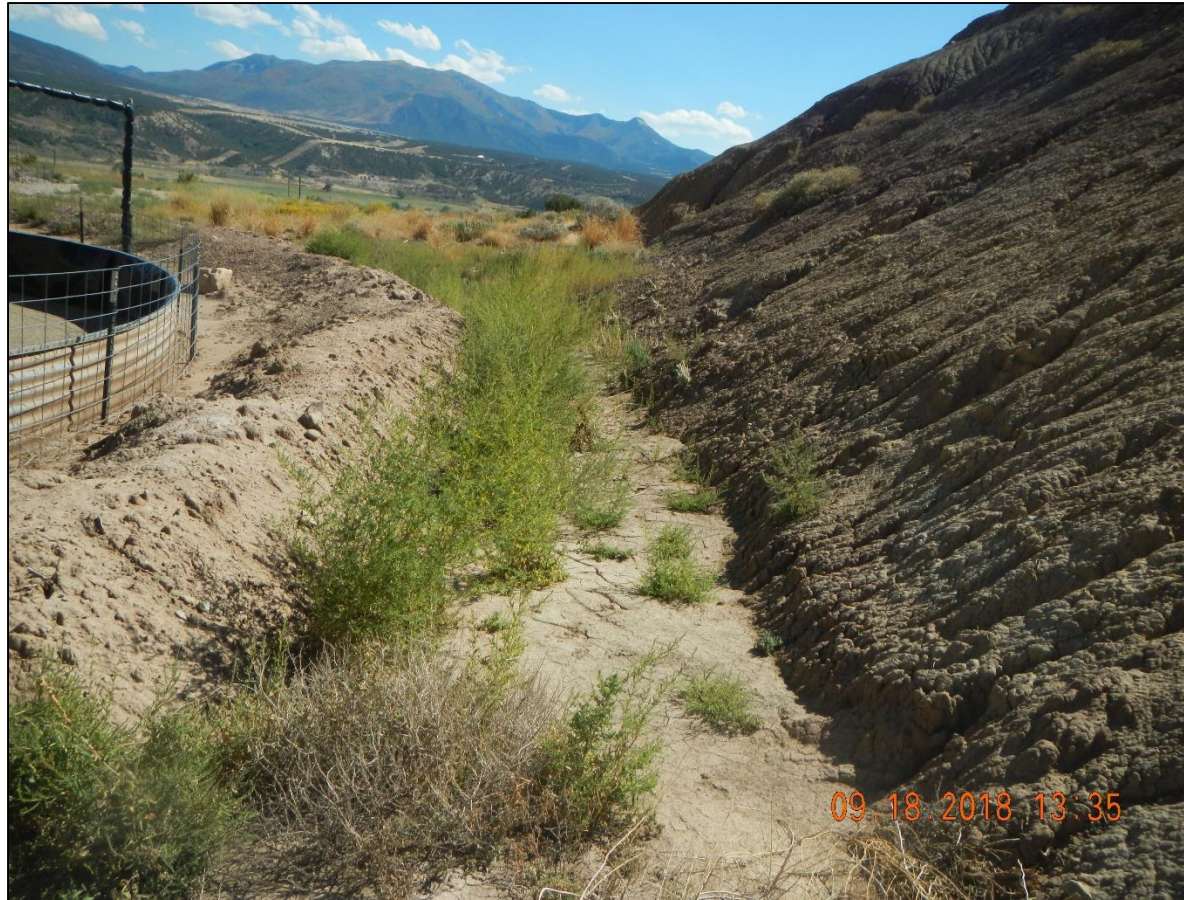
Sediment build up and dead weed debris in ditch behind tank battery.
