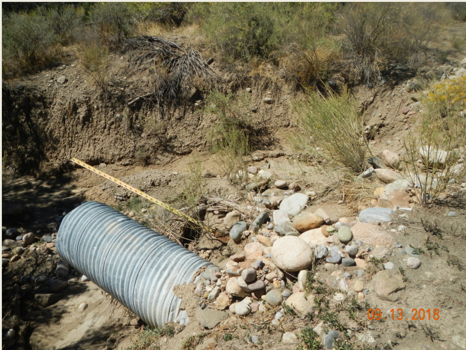
Photo 4. View of erosion at culvert outlet where culvert is blocked on upstream side and stormwater flows over the road surface resulting in erosion on the road and where it flows into the drainage around the culvert.
