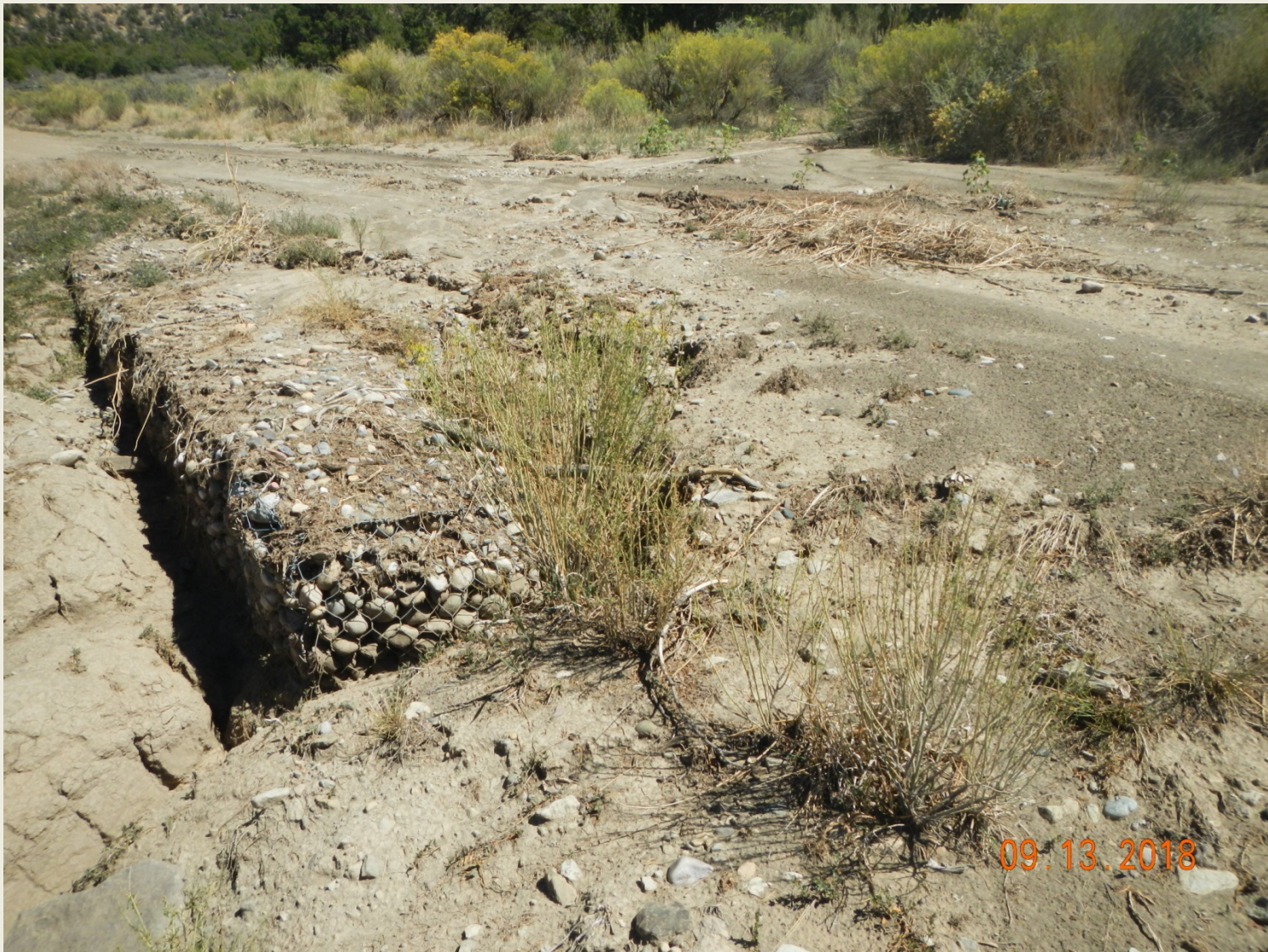
Photo 7. View of area along the access road, downstream from photos 4-6, where drainage crosses the access further from the well pad. Stormwater flows over and erodes the access road and cut-banks. Upstream culvert inlet not observable.
