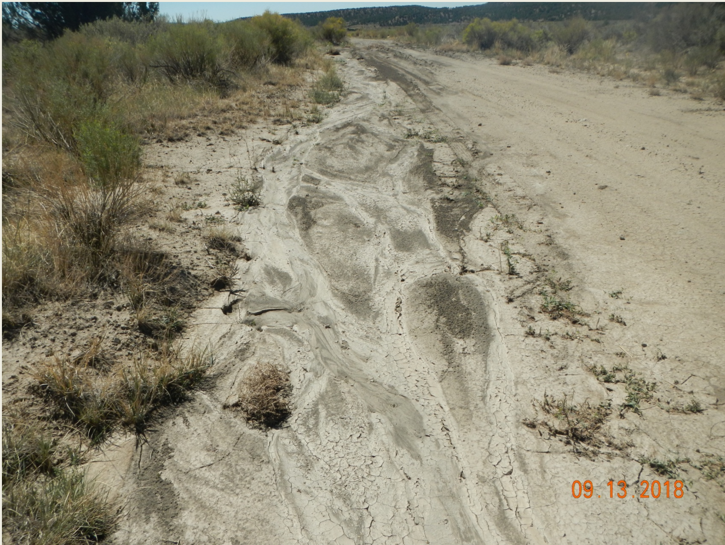
Photo 6. View of area on the access road where roadside ditches are not present/functining and stormwater flows along the road eroding the road and depositing sediment.
