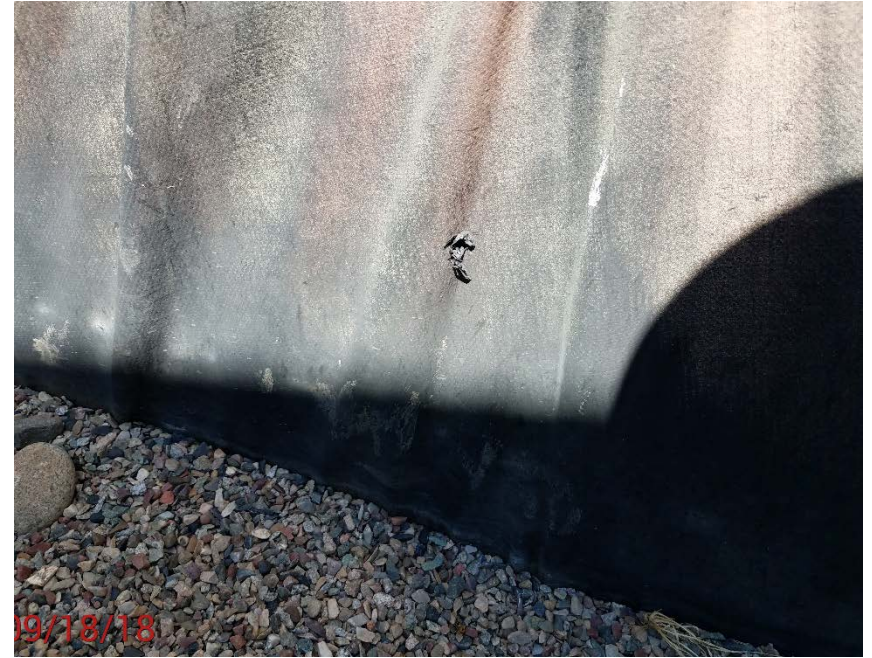
Location Photo #4, hole in liner near stairs
