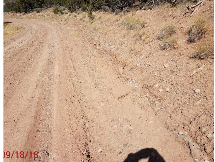
Location Photo #6, Heavy erosion along access road.
