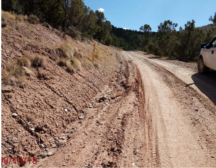
Location Photo #5, Heavy erosion along access road
