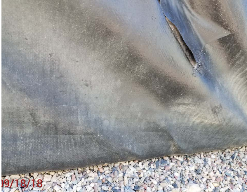
Location Photo #3, patch faild
