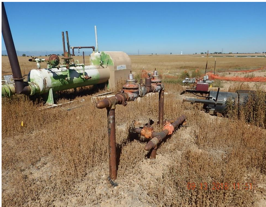
Unused equipment; disconnected horizontal separator, unused ECD (vent stack) and unmarked flowline risers.
