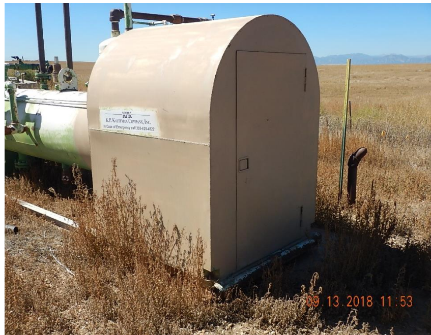
Unused flowline riser near the NW corner of horizontal separator; not marked or locked/ tagged out.
