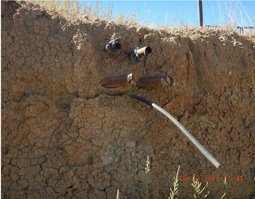
Close up view of flowlines exposed in excavation; Fiberglass, carbon steel and poly flowlines of numerous sizes were encountered during excavation. Some cut ends have been covered with tape (not an acceptable means of sealing ends)
