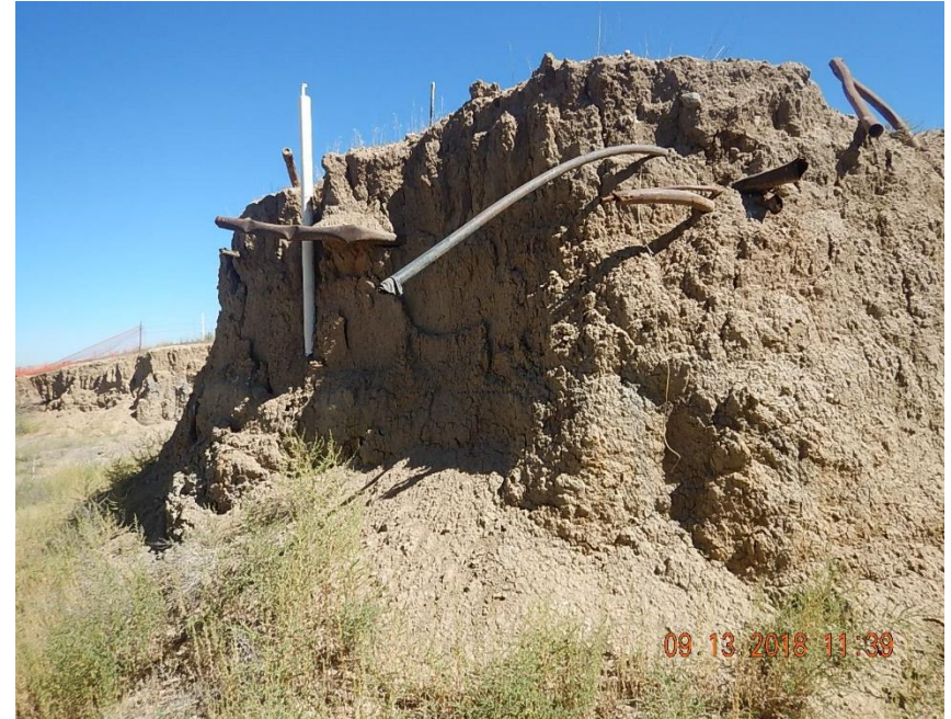
View of inactive flowlines exposed along the north side of the excavation. Flowlines have not been located or marked on surface (adjacent to excavation). Flowlines (exposed to surface as risers) have not been abandoned per rule 1105.
