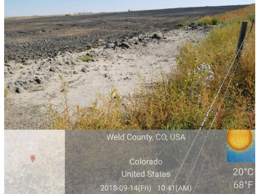
Photo 8. Sediment filled perimeter berm on west side of location
