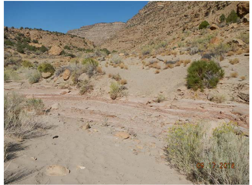
Photo 6: Access road washed out at crossings of natural drainages.
