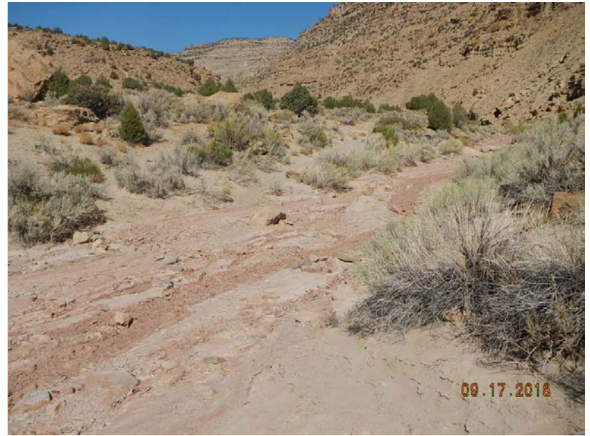
Photo 8: Access road washed out at crossings of natural drainages.
