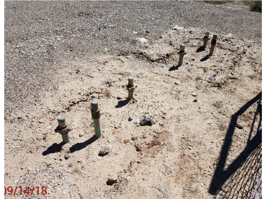
Location Photo #4, unmarked/unused flowline risers.
