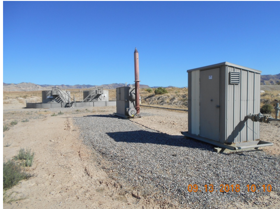
Meter housing, Separator and Tank Battery
