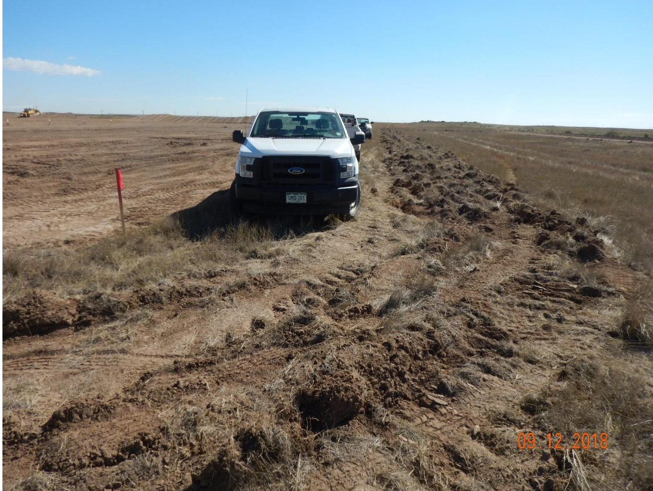
Photo 1: Photo taken from the southwest corner of the location, facing east. Photos 1-3 provide overview of the construction in process. Photo also shows operator implemented surface roughening along perimeter of the location. Surface roughening is a temporary erosion control BMP that needs to be used in conjunction with other BMPs.
