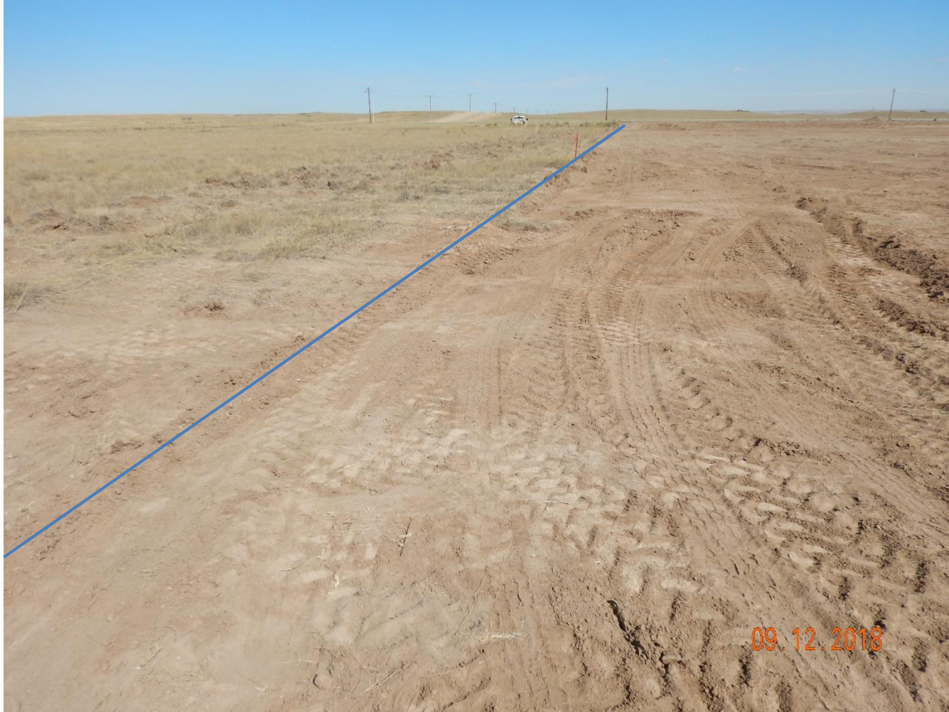
Photo 16: Photo taken from the west end of the location, facing north. Photo shows the pad and the adjacent lands. It does not appear as though sufficient topsoil salvage has been conducted on this area of the pad.
