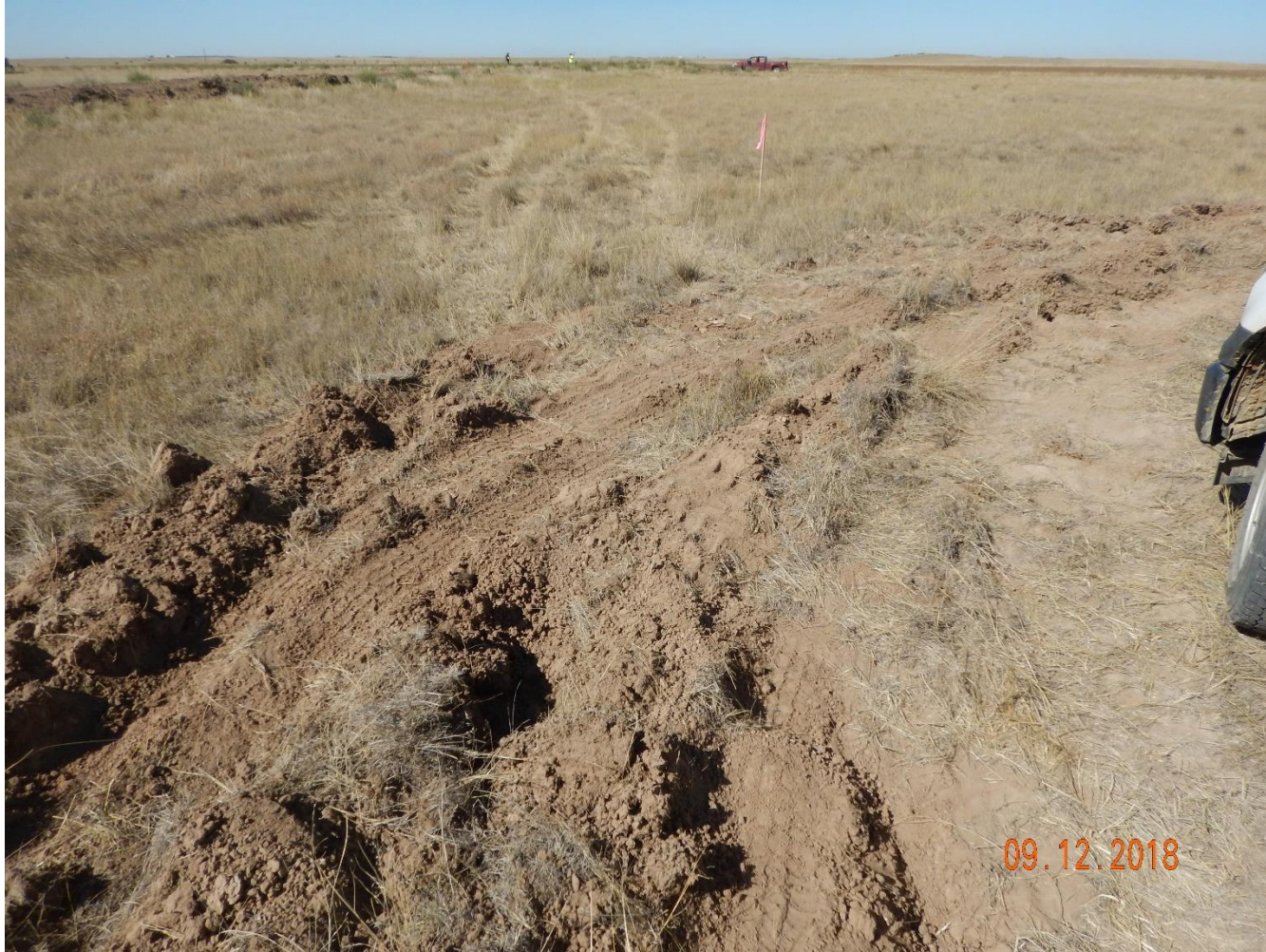
Photo 4: Photo taken from the southwest corner of the location, facing west. Photo shows surface roughening appears to have been traveled over by vehicle traffic rendering the control to no longer be in proper functioning condition.
