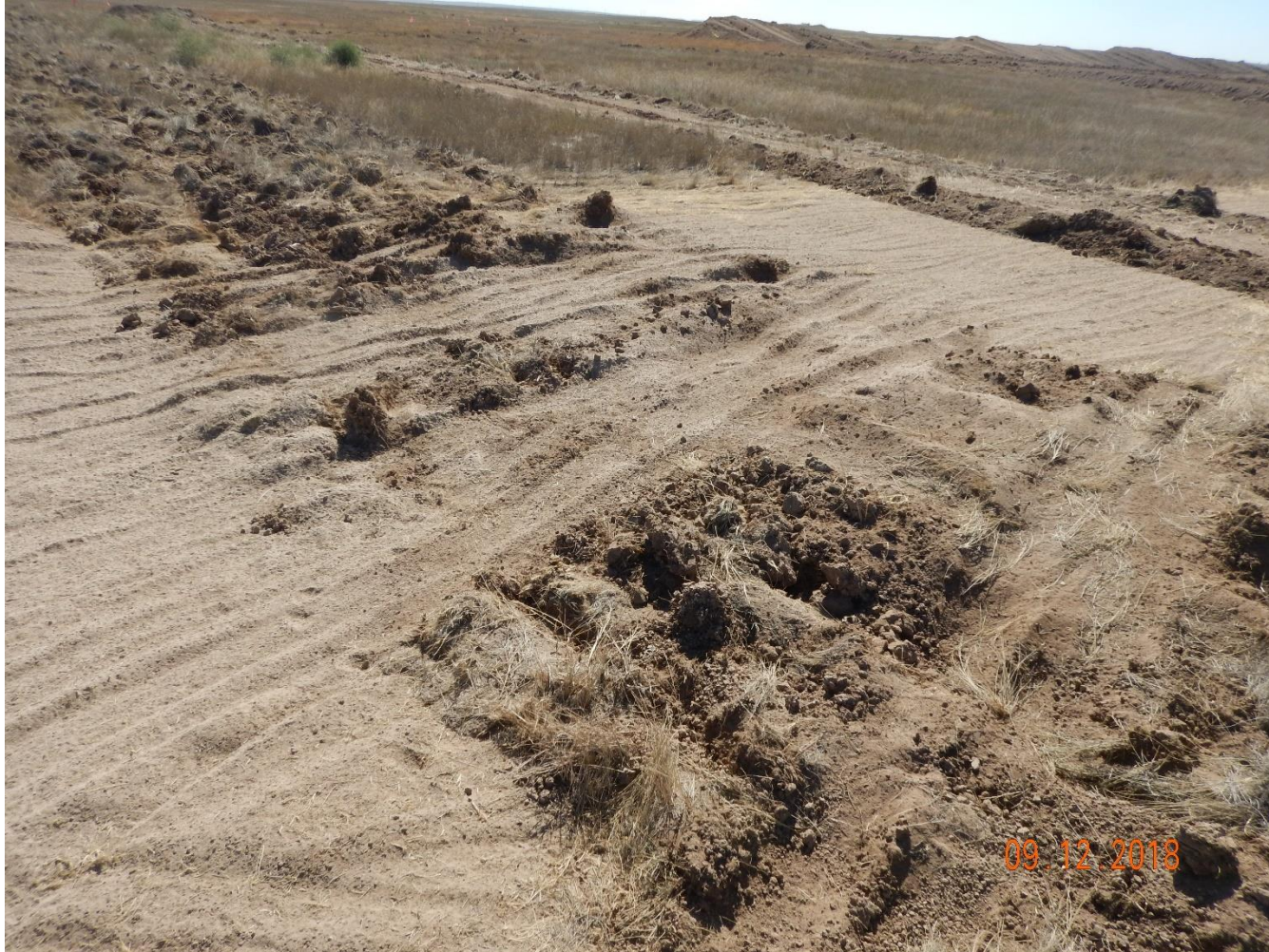
Photo 9: Photo taken from the north end of the location, facing southeast. Photo shows surface roughening appears to have been traveled over by vehicle traffic rendering the control to no longer be in proper functioning condition.
