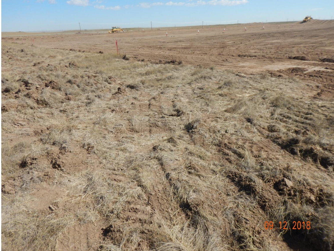
Photo 6: Photo taken from the west end of the location, facing northeast. Photo shows surface roughening appears to have been traveled over by vehicle traffic rendering the control to no longer be in proper functioning condition.
