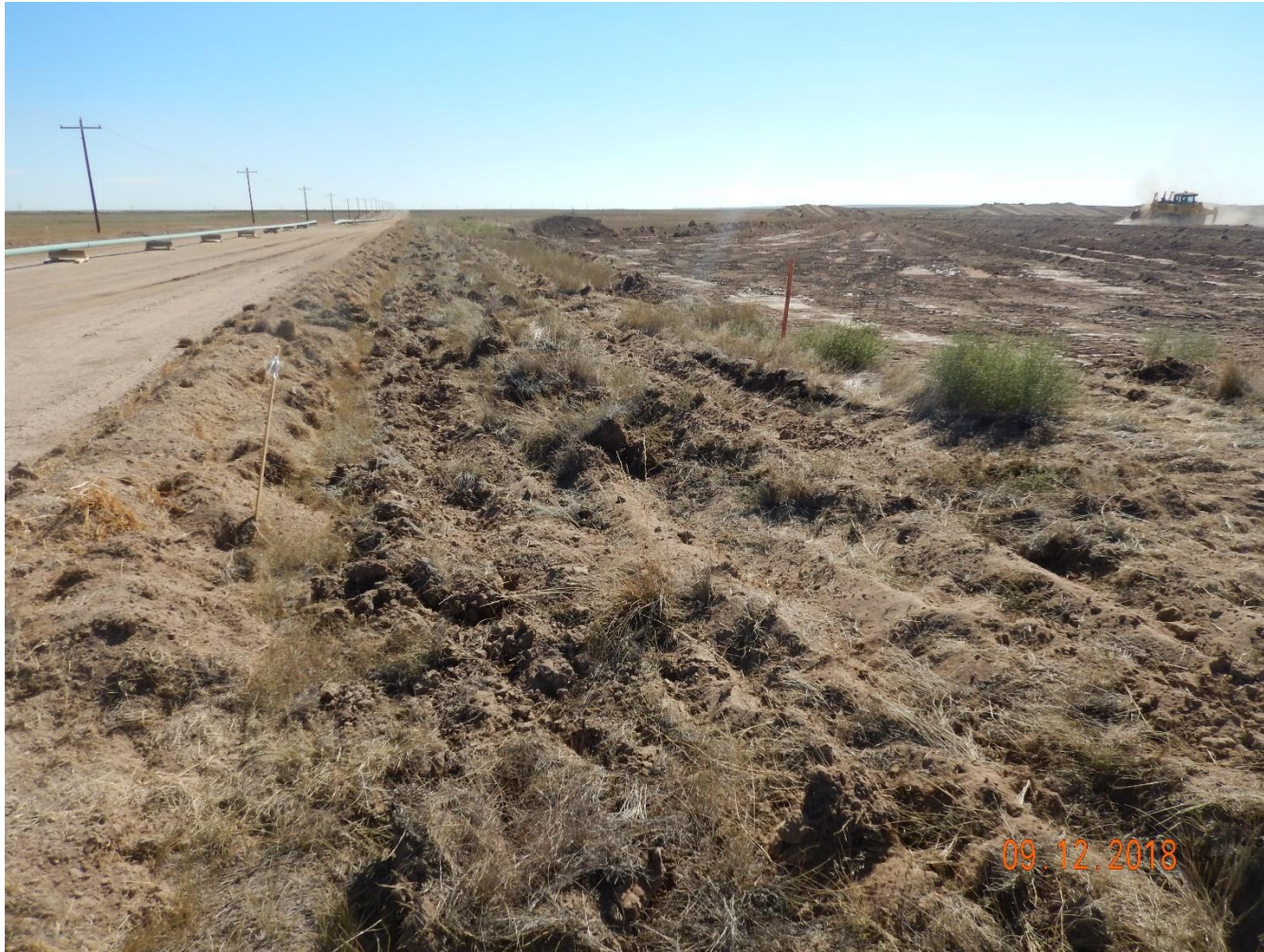
Photo 8: Photo taken from the northwest corner of the location, facing east. Photo also shows operator implemented surface roughening along perimeter of the location. Surface roughening is a temporary erosion control BMP that needs to be used in conjunction with other BMPs.
