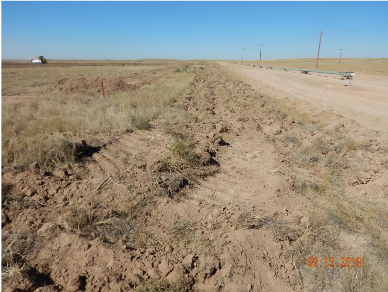
Photo 12: Photo taken from the northeast corner of the location, facing west. Photo also shows operator implemented surface roughening along perimeter of the location. Surface roughening is a temporary erosion control BMP that needs to be used in conjunction with other BMPs.
