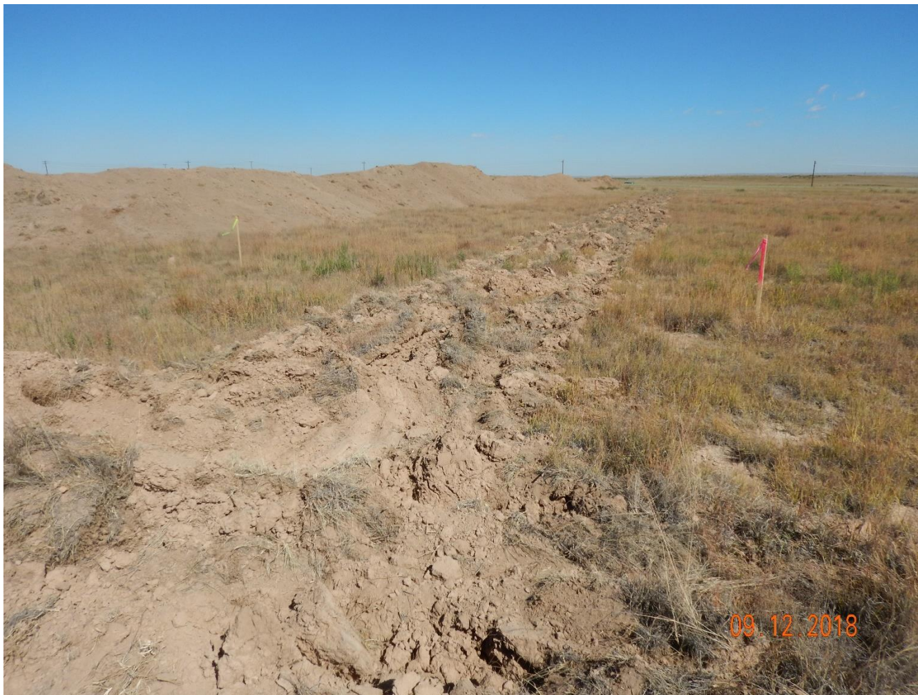
Photo 13: Photo taken from the southeast corner of the location, facing north. Photo also shows operator implemented surface roughening along perimeter of the location. Surface roughening is a temporary erosion control BMP that needs to be used in conjunction with other BMPs.
