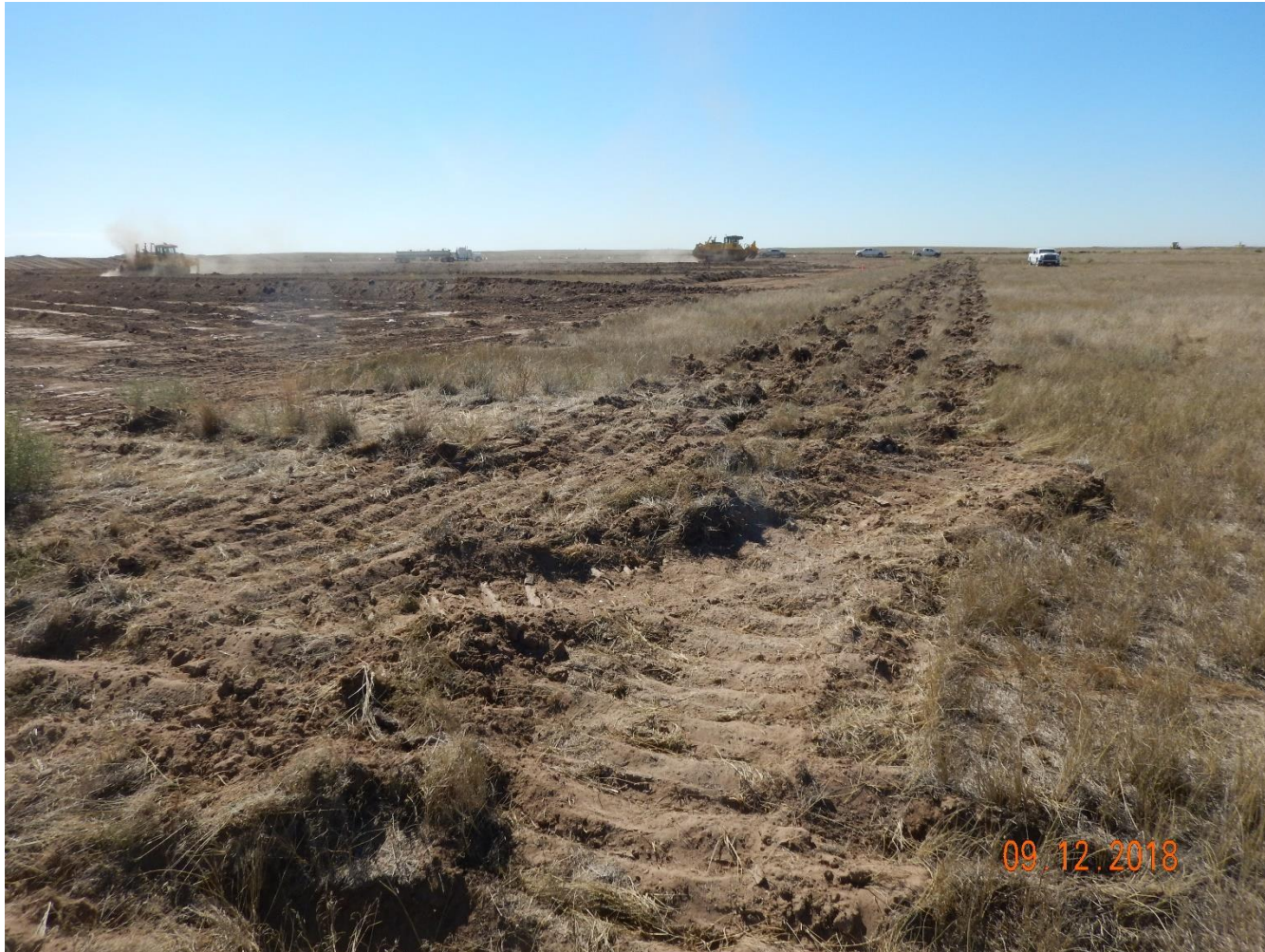
Photo 7: Photo taken from the northwest corner of the location, facing south. Photo also shows operator implemented surface roughening along perimeter of the location. Surface roughening is a temporary erosion control BMP that needs to be used in conjunction with other BMPs.
