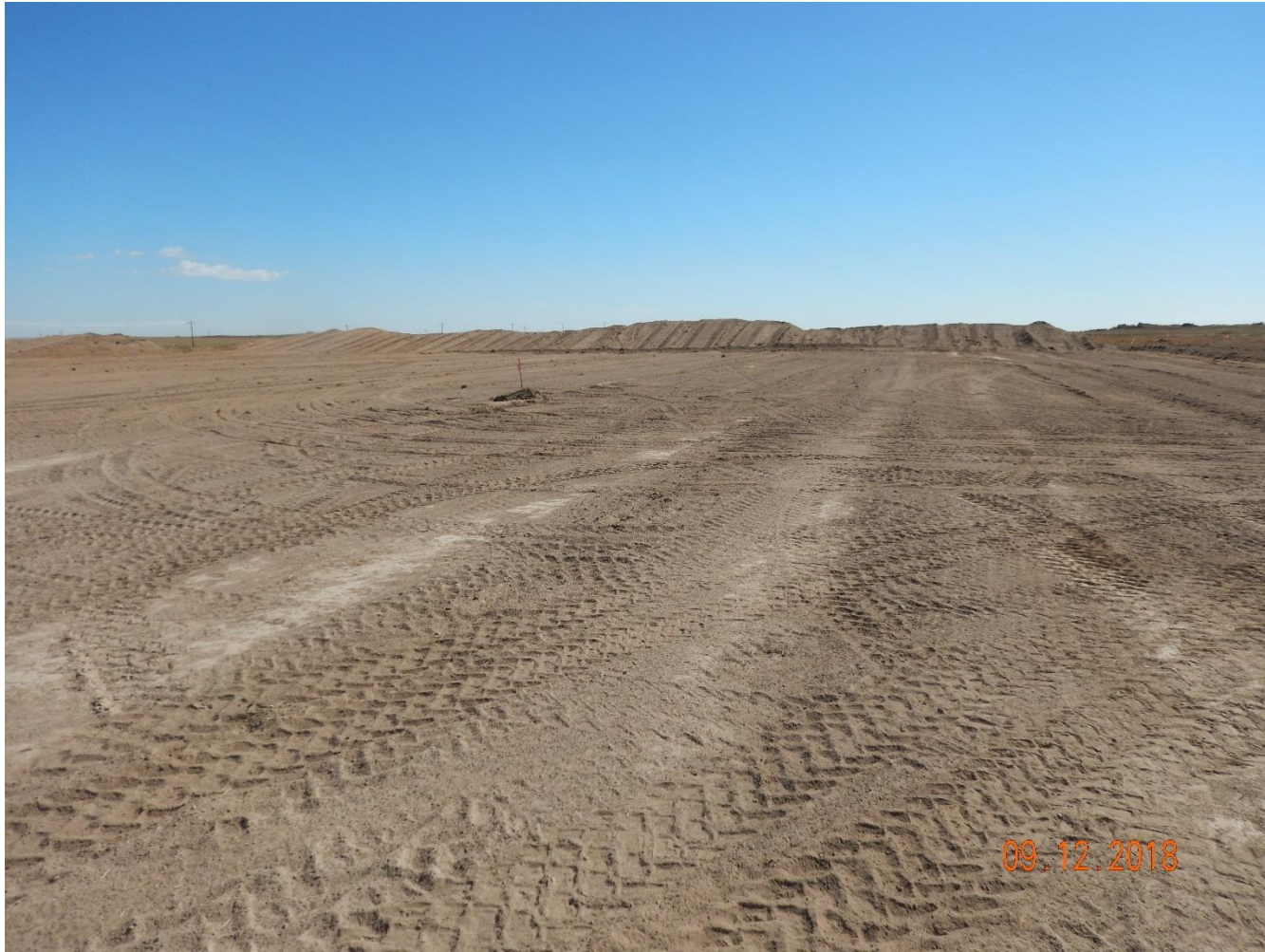
Photo 15: Photo taken from the pad, facing east. Photo shows what appears to be the topsoil stockpile on the location. Soil salvage currently in process, however, there are areas where topsoil remains evident that the contractor has indicated to be “at grade”.
