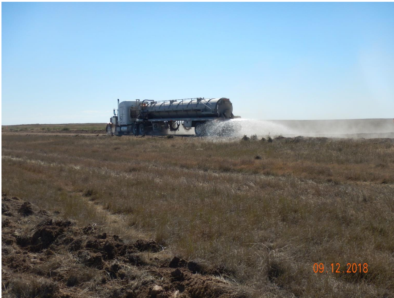
Photo 5: Photo showing actively spraying road with water to mitigate dust
