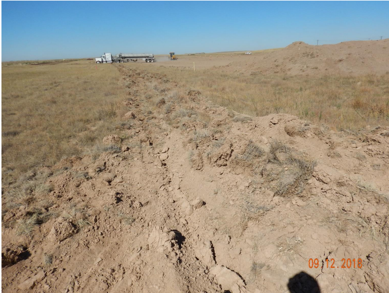
Photo 14: Photo taken from the southeast corner of the location, facing west. Photo also shows operator implemented surface roughening along perimeter of the location. Surface roughening is a temporary erosion control BMP that needs to be used in conjunction with other BMPs.
