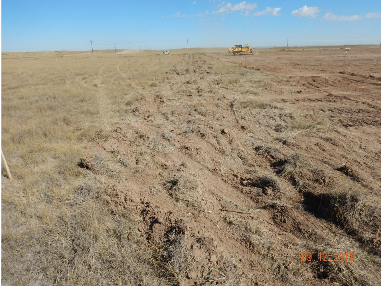
Photo 3: : Photo taken from the southwest corner of the location, facing north. Photos 1-3 provide overview of the construction in process. Photo also shows operator implemented surface roughening along perimeter of the location. Surface roughening is a temporary erosion control BMP that needs to be used in conjunction with other BMPs.
