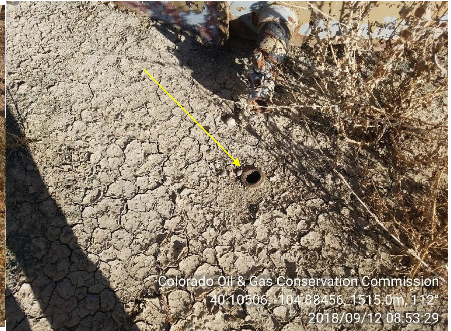
Photo 4. Unmarked unused riser/no lock out tag out
