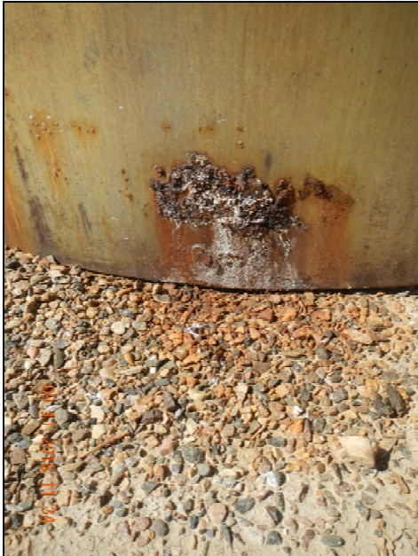
Photo 3. Corrosion on tank.
