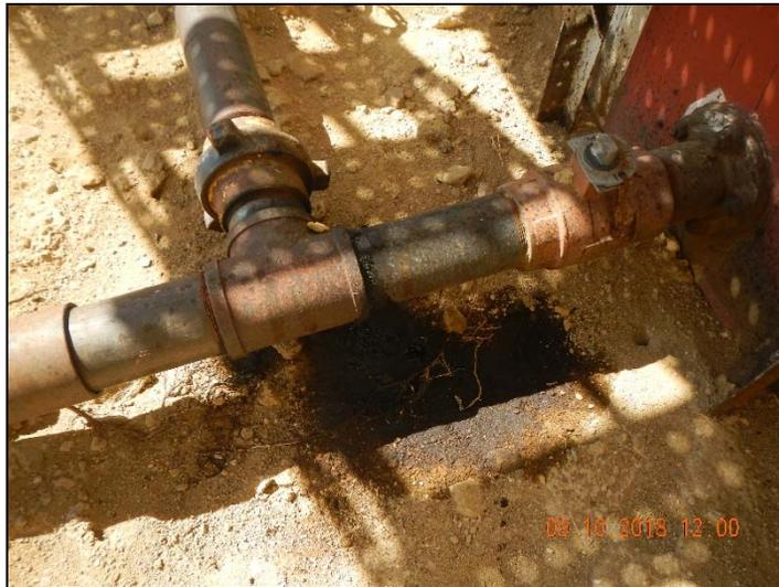
**Photo 9. Stained soil at tank connection.**
