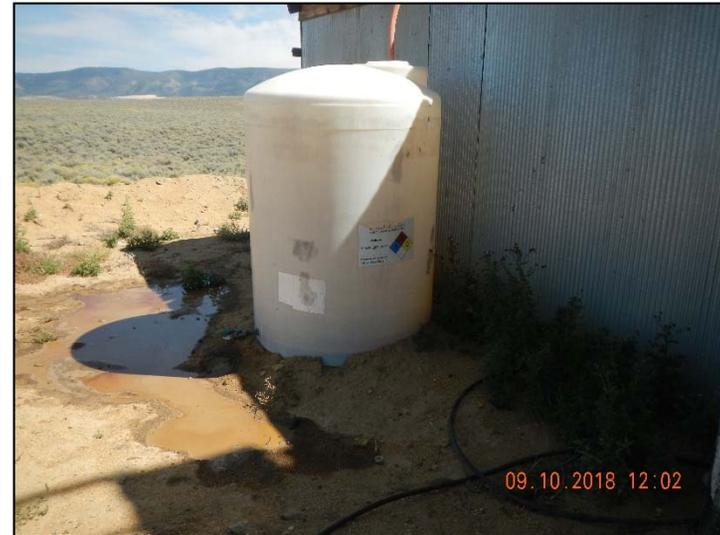
Photo 14. Apparent Methanol spill.
