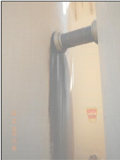
Photo 11. Staining down tank side.
