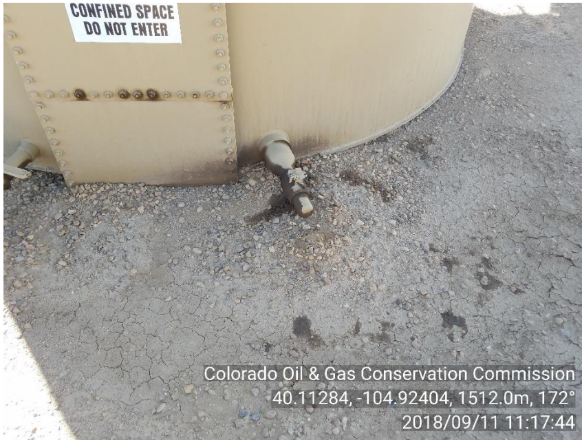
Photo 5. Staining on valve and soil on west crude oil tank.
