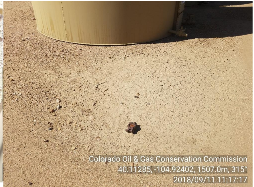
Photo 4. Unmarked unused riser southeast of east crude oil tank.
