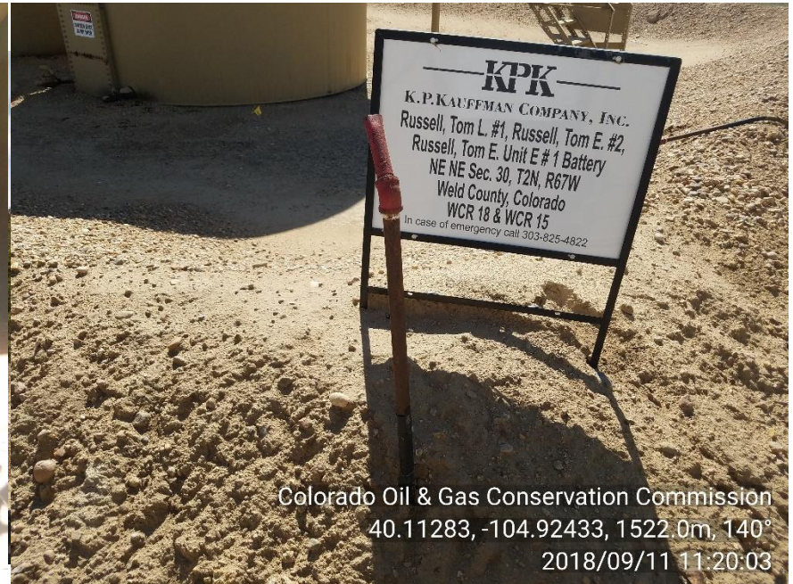
Photo 8. Unmarked unused riser near tank battery sign.
