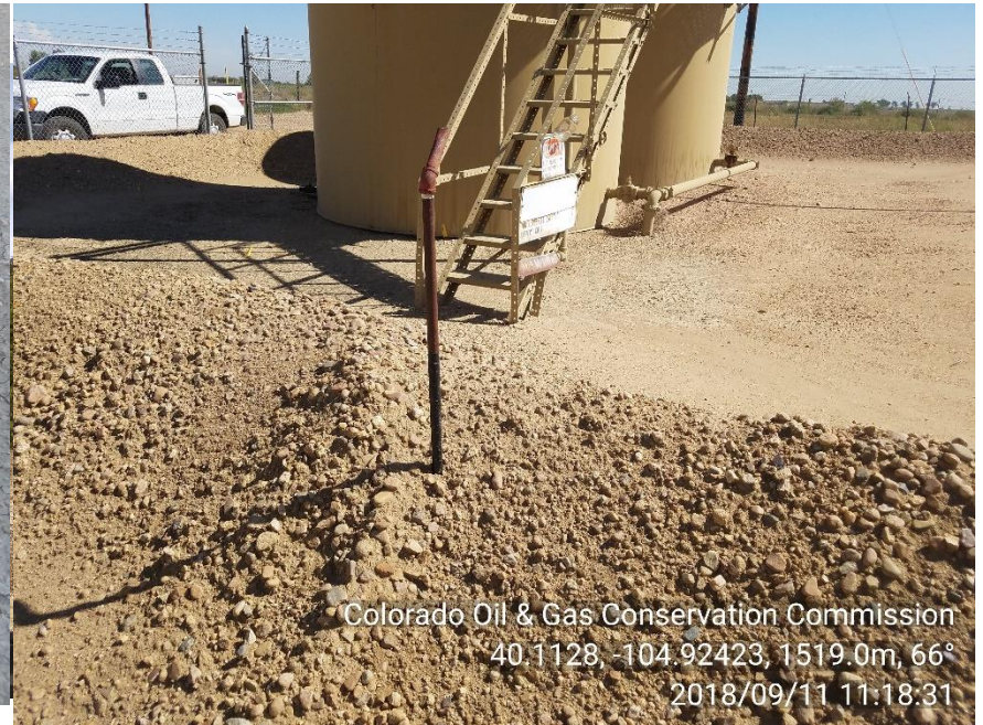
Photo 6. Unmarked unused riser southwest of west crude oil tank.
