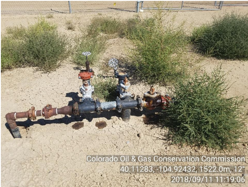
Photo 7. Leaking valve on riser west of heated separators.
