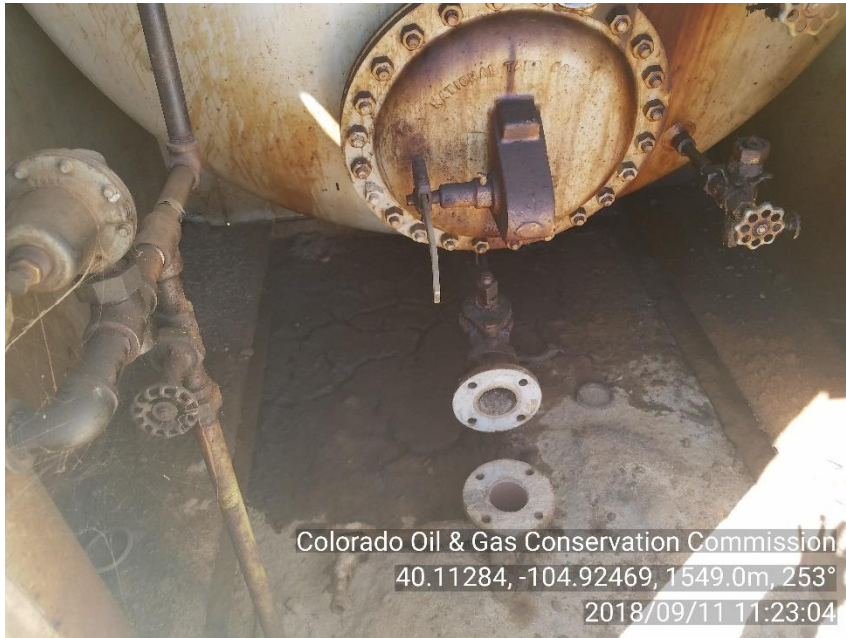
Photo 9. Stained soil under north heated separator
