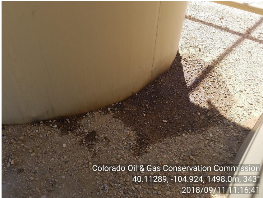
Photo 3. Stained soil near west edge of east crude oil tank.
