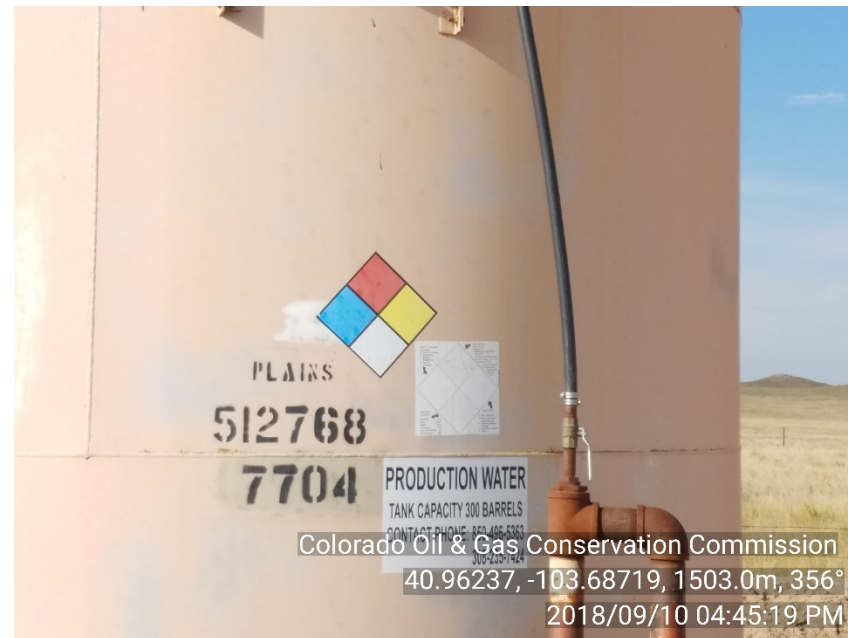
Photo #13 USA 21-6 Produced H2O tank NFPA placard numbers illegible
