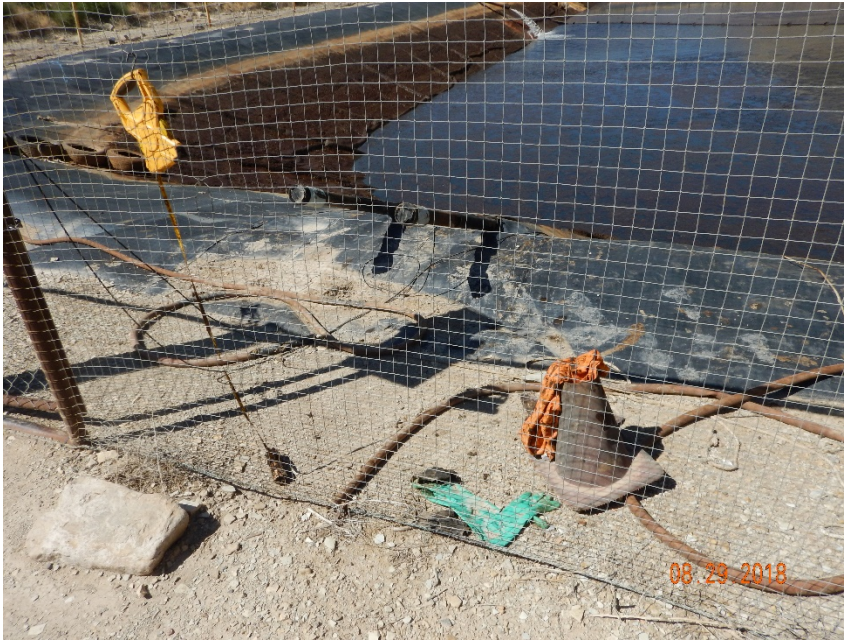
Photo #9 – Oily rag, gloves, hose, and cone stored inside of pit mesh. Note sediment encroaching on pit liner from south.
