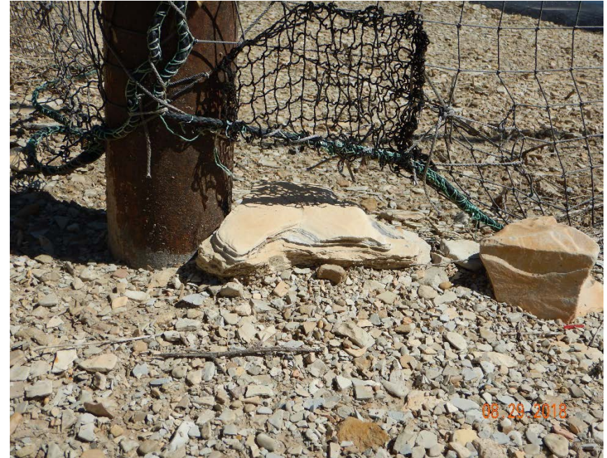
Photo #4 – Gap in base of mesh at NW corner of pit is large enough to provide wildlife access.
