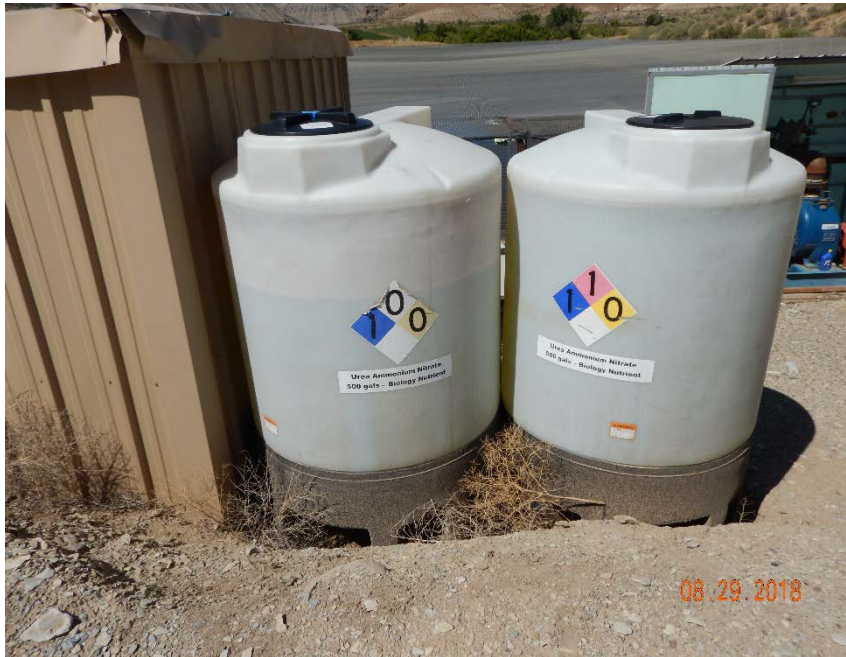
Photo #11 – Urea Ammonium Nitrate containers stored south of pit lack secondary containment device.
