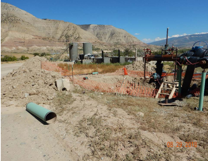
Photo #19 – Flowline excavation located at entrance to location.
