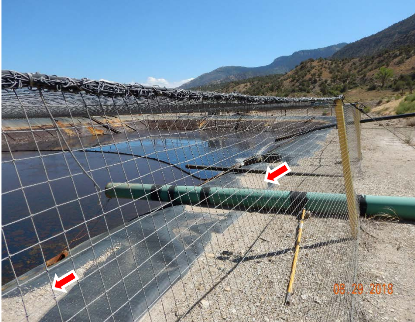
Photo #7 – Discharge pipelines from tank battery on west side of pit are in direct contact with pit liner. Note angular rocks encroaching on pit liner (red arrows).
