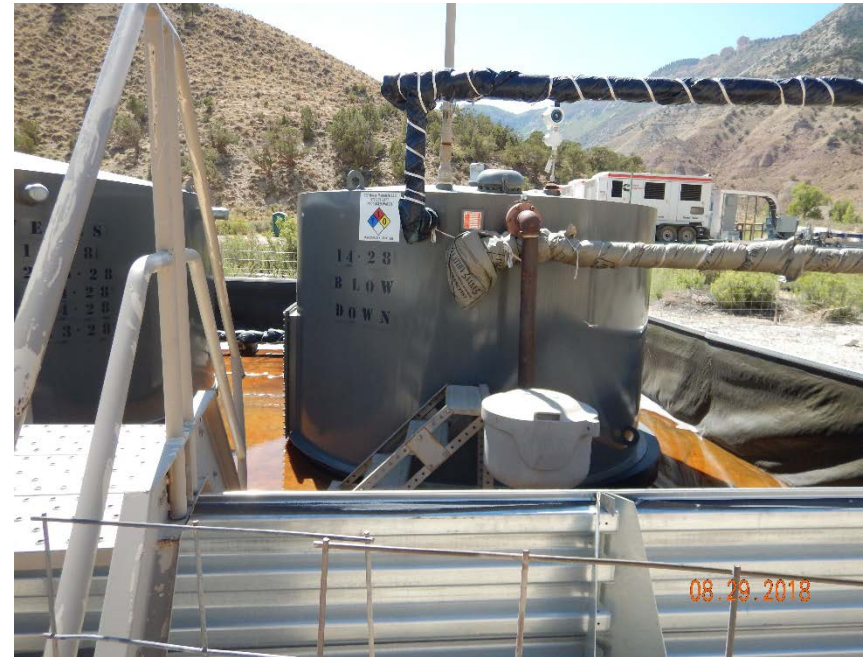
Photo #18 – 80 bbl produced water tank located southwest of pit.
