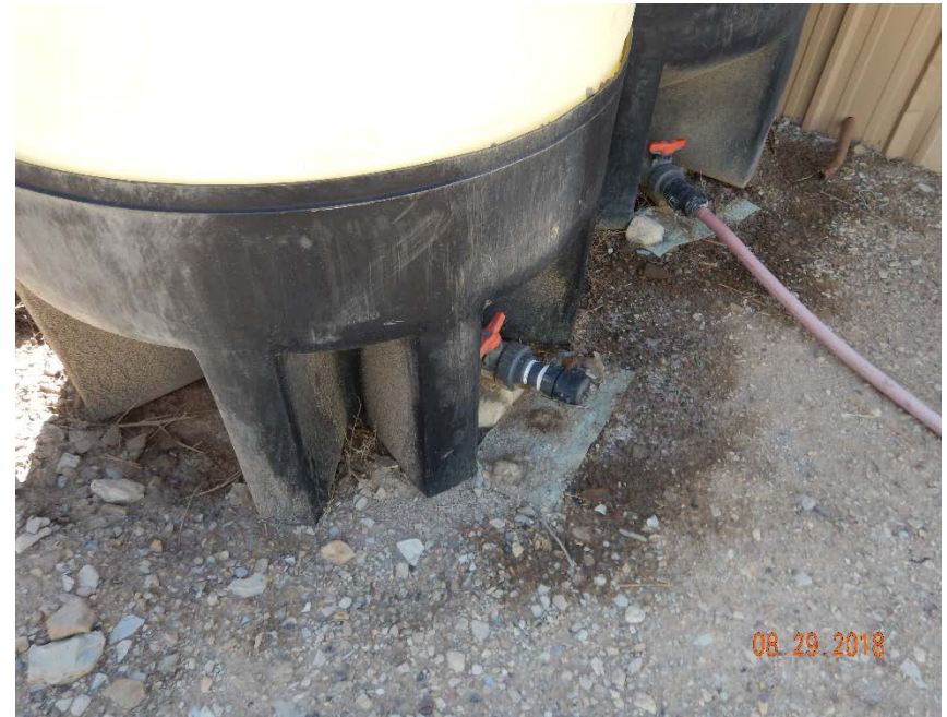
Photo #12 – Historical accumulation of impacted soil underlying chemical storage containers from previous photo.
