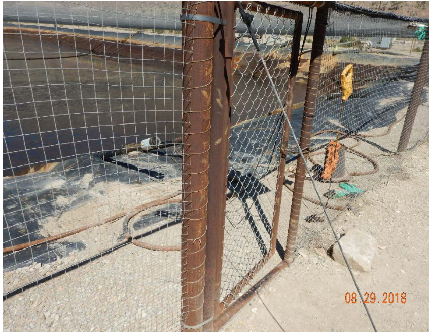
Photo #3 – Second gate located at SW corner of pit provides access to leak detection system. Note that gap between gate and post is big enough to provide wildlife access. Angular rocks encroaching upon pit liner.
