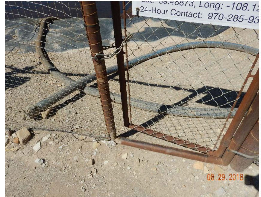
Photo #2 - Gap between gate and post is large enough to grant wildlife access.
