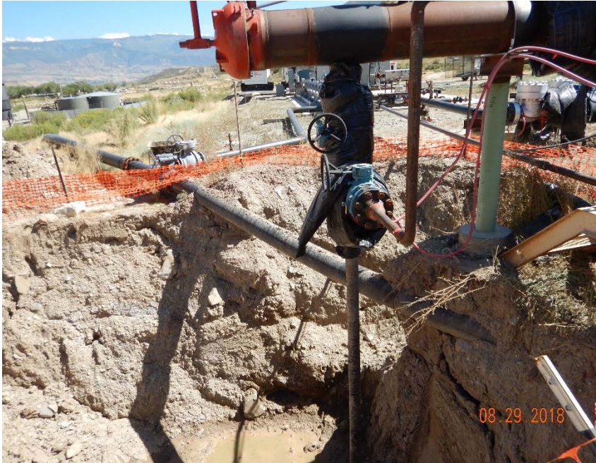
Photo #21 – Flowline suspended across flowline excavation.
