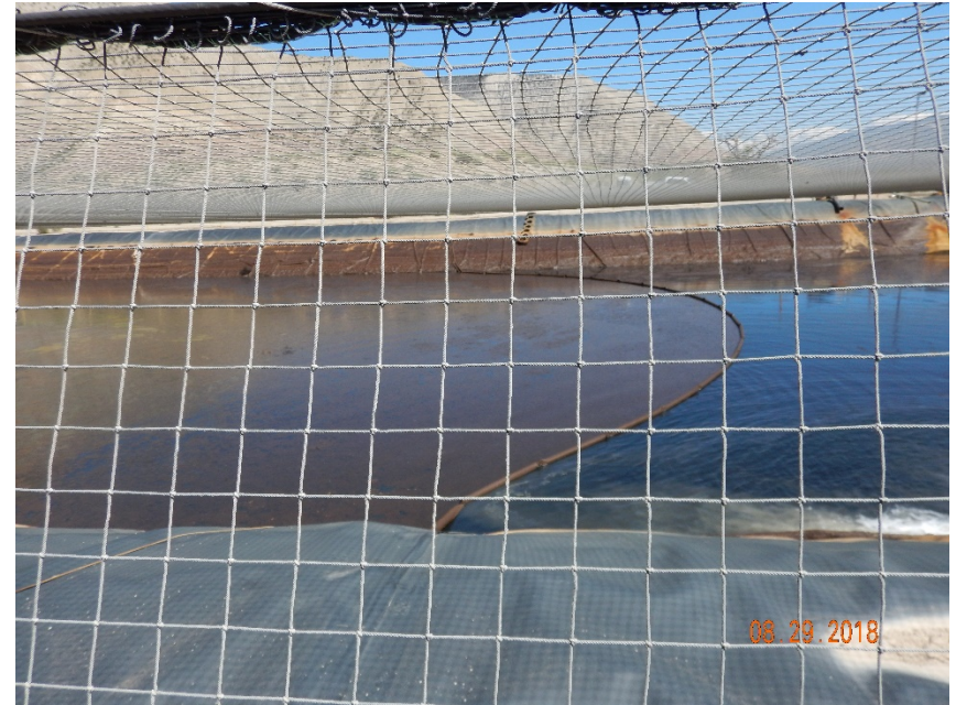
Photo #8 – Free product visible on fluid surface on both sides of boom, as well as liner.
