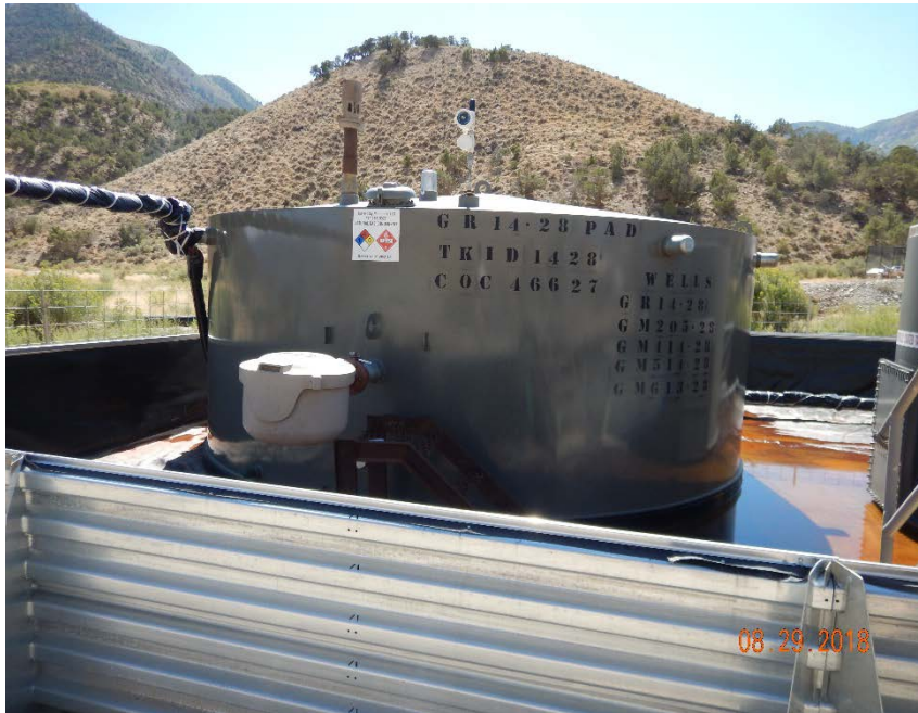
Photo #17 – 200 bbl condensate AST located southwest of pit.
