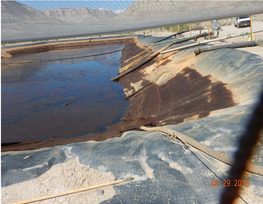
Photo #5 – Multiple discharge hoses and pipes along SE corner of pit are in direct contact with pit liner.
