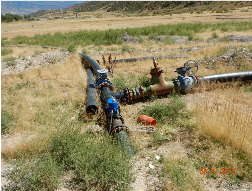
Photo #13 – T-intersection in surface pipeline located SE of pit.
