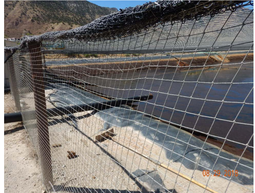
Photo #6 – Multiple discharge pipes along south end of pit are in direct contact with pit liner.
