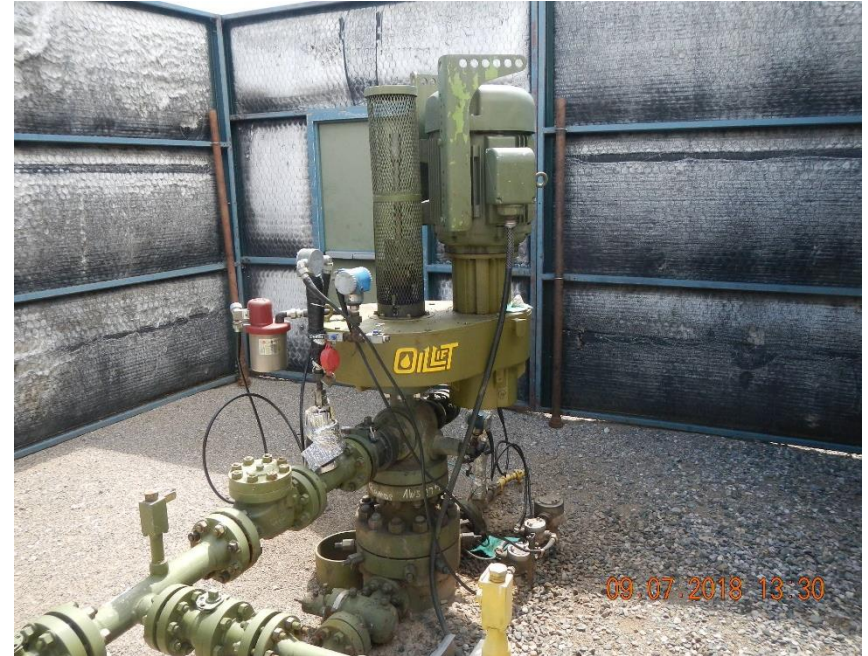
Neva Dove A #2 well head and progressive cavity pump. Pump is leaking oil.
