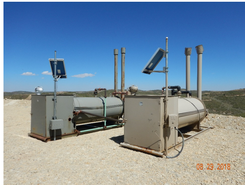
Photo #8 – Unused separators located north of pit.
