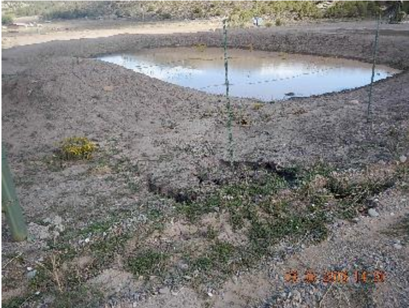
Photo 7: Rilling and erosion channeling at access road entry point.
