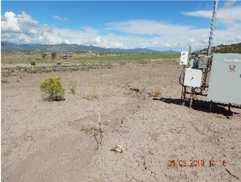
Photo 5: Erosion channel off NE fill slope.
