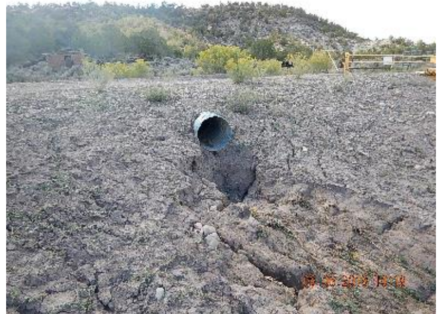
Photo 6: Erosion on outflow side of culvert into sediment retention pond.
