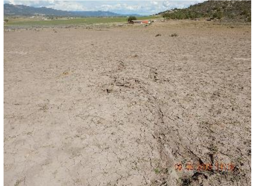
Photo 4: Erosion channel off NE fill slope.
