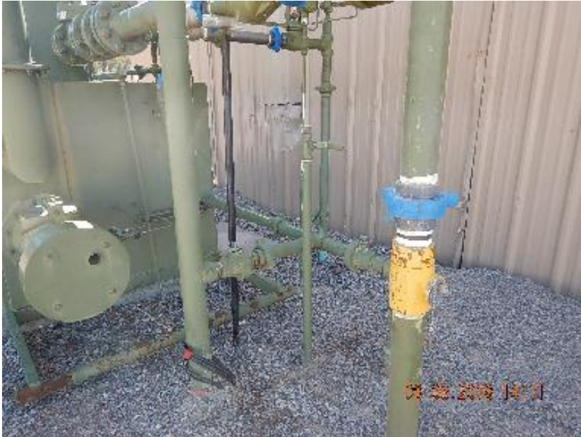
Photo 3: Steel 1" riser (A) point at separator.
