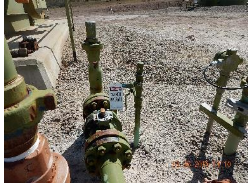
Photo 2: Locked out, tagged, and plugged 1" (B) point riser at wellhead.
