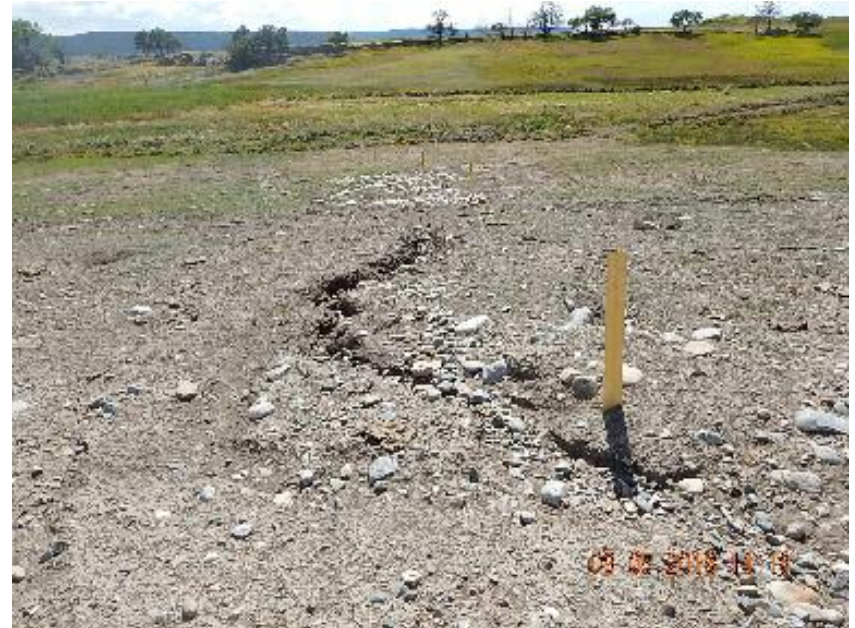
Photo 4: Erosion channel on W fill slope.
