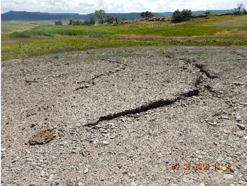
Photo 3: Erosion channel on W fill slope.
