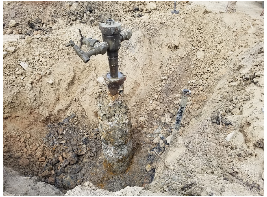
Photo 2. Excavation around wellhead.
