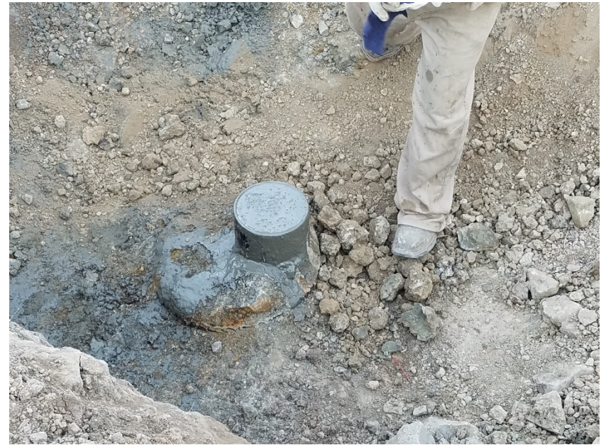
Photo 4. Cement to surface.
