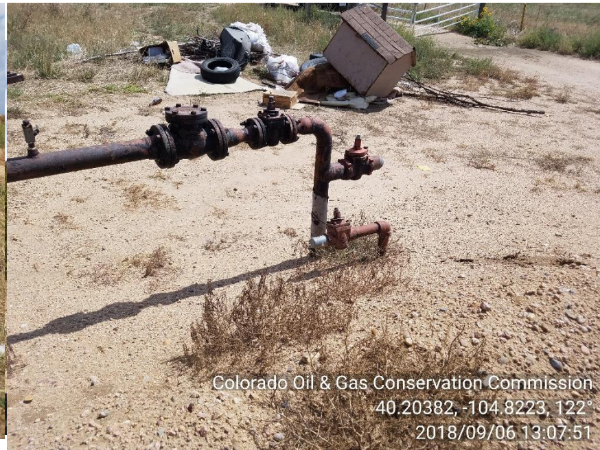
Photo 6. Unused unmarked riser near meter at tank battery
