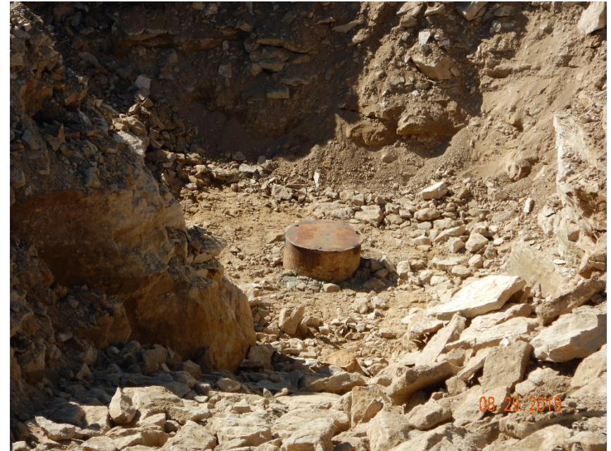
Photo #4 – Unidentified well casing with welded cap is located in center of excavation.
