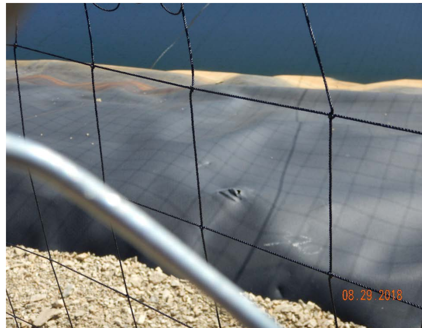
Photo #8 – Hole in liner observed on west pit berm.
