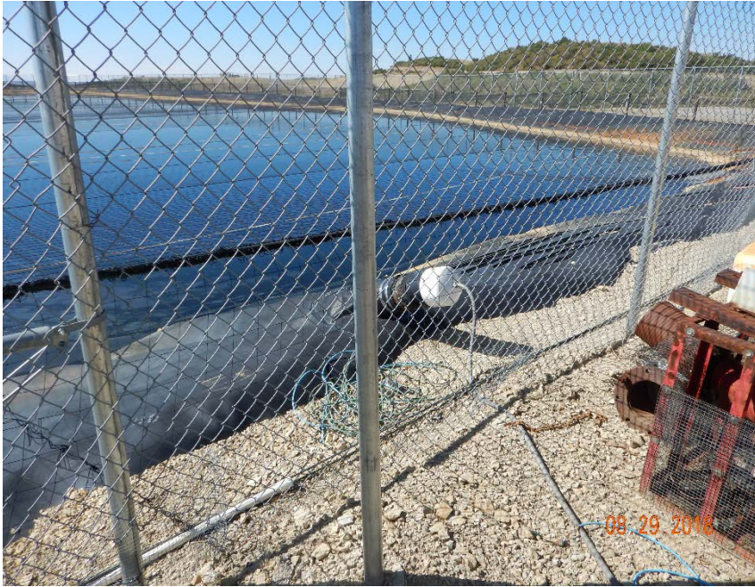
Photo #11 – Leak detection system on north side of pit.
