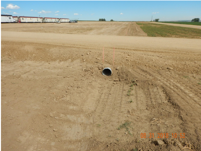
Photo 1. Photo taken from the entrance of the well location, facing North. Vehicle tracking pad was observed at the intersection of CR42. Ditch and berm BMP has been installed around the entire perimeter of the location in conjunction with other BMPs.
