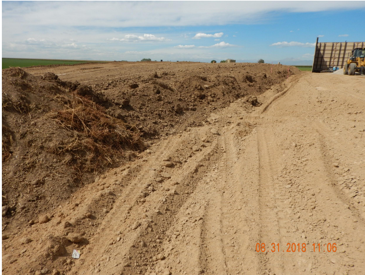
Photo 7. Photo taken from the eastern topsoil stockpile, facing West. Topsoil has been salvaged and stored along the southern location. However, topsoil has not been stabilized and drilling operations are underway.
