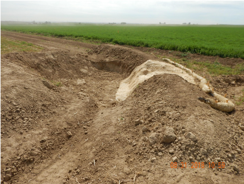
Photo 3. Photo taken from the southwest sediment trap, facing South. Sediment trap has been installed with an outlet protection device but no inlet protection.
