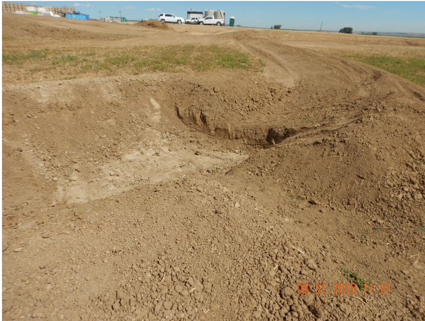
Photo 5. Photo taken from the southern sediment trap, facing North. Appears this was designed to be a sediment trap because of the outfall, but has not been completed.
