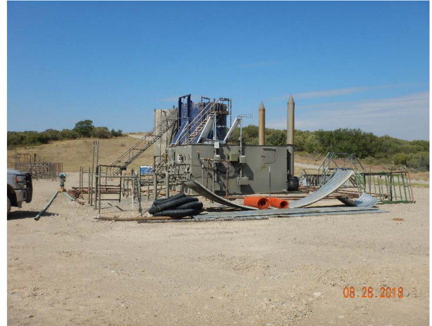
Photo #2 – Metal tank battery berm components have been removed as part of Remediation Project #11621.
