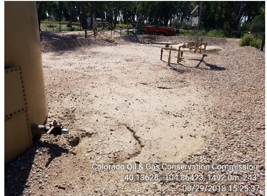
Rear of tank (areas of subsidence)
