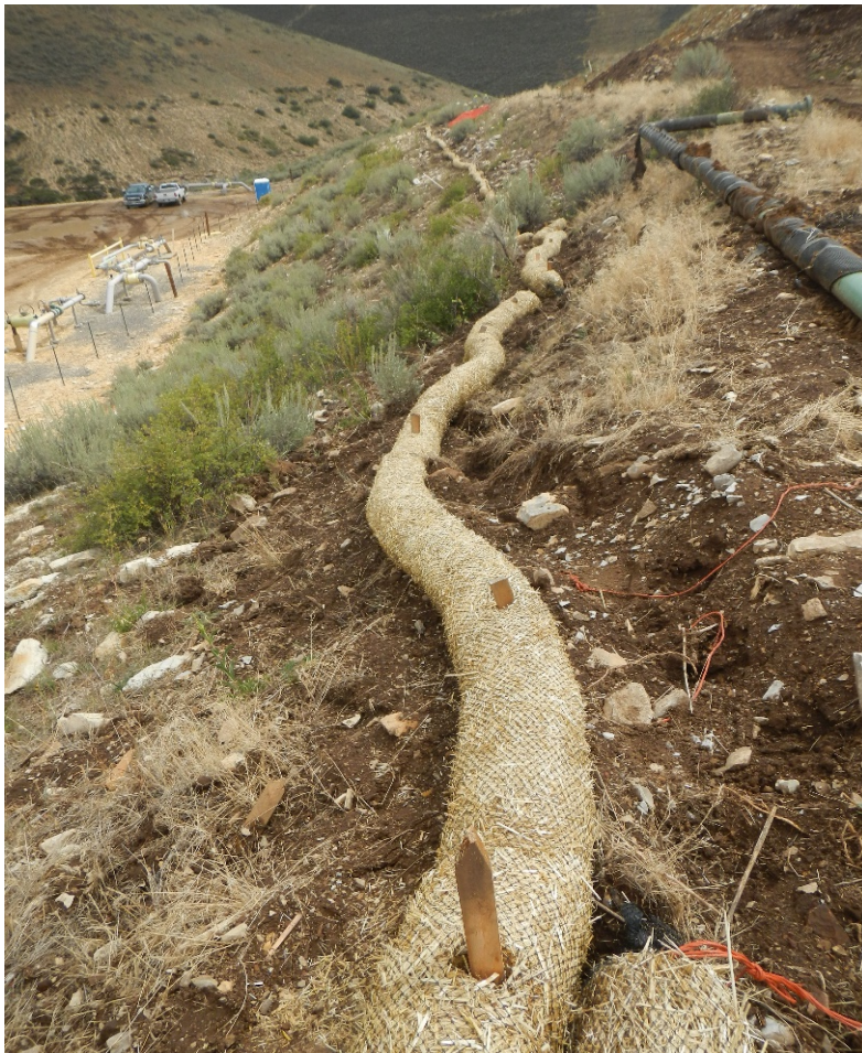
Photo#5: BMPs have been installed around Location Perimeter
