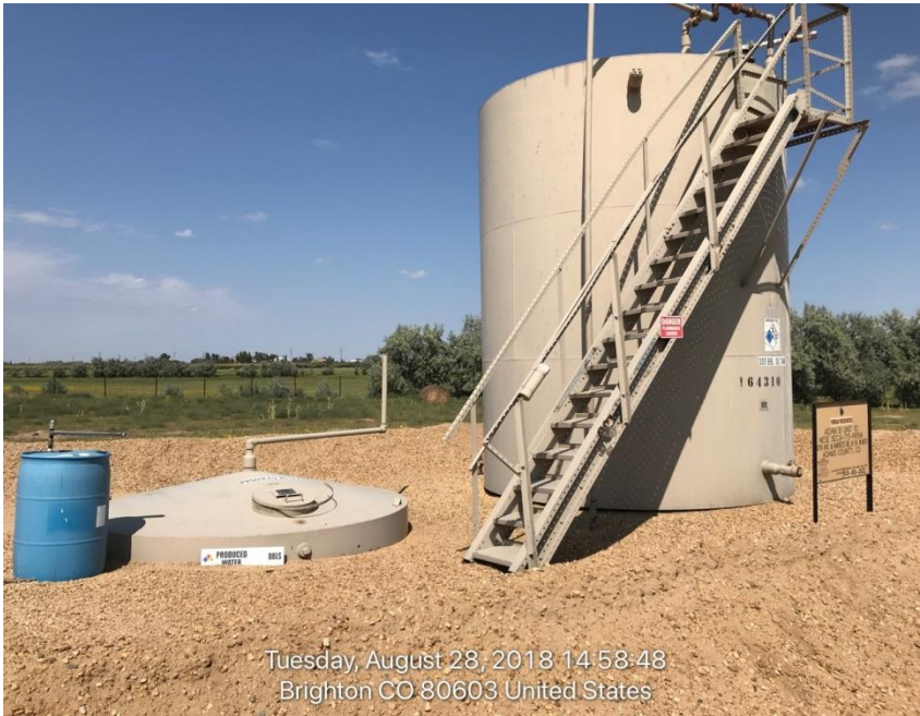
Photo#1 Production tank and produced water pit
