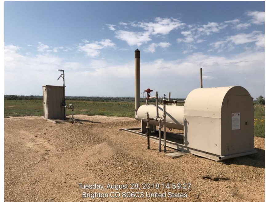
Photo#2 Separator and gas meter
