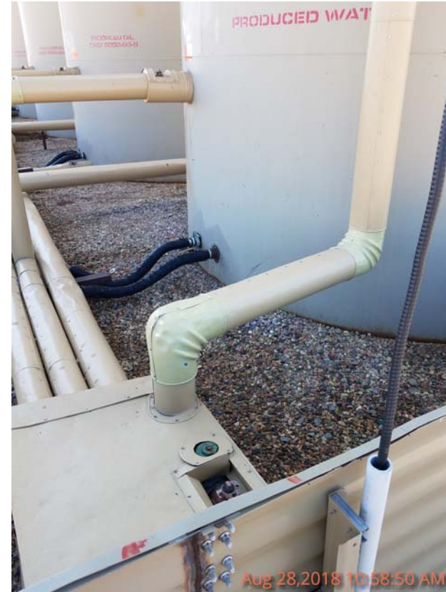
Photo 5 – Piping entering produced water tank, piping valves appear open.
