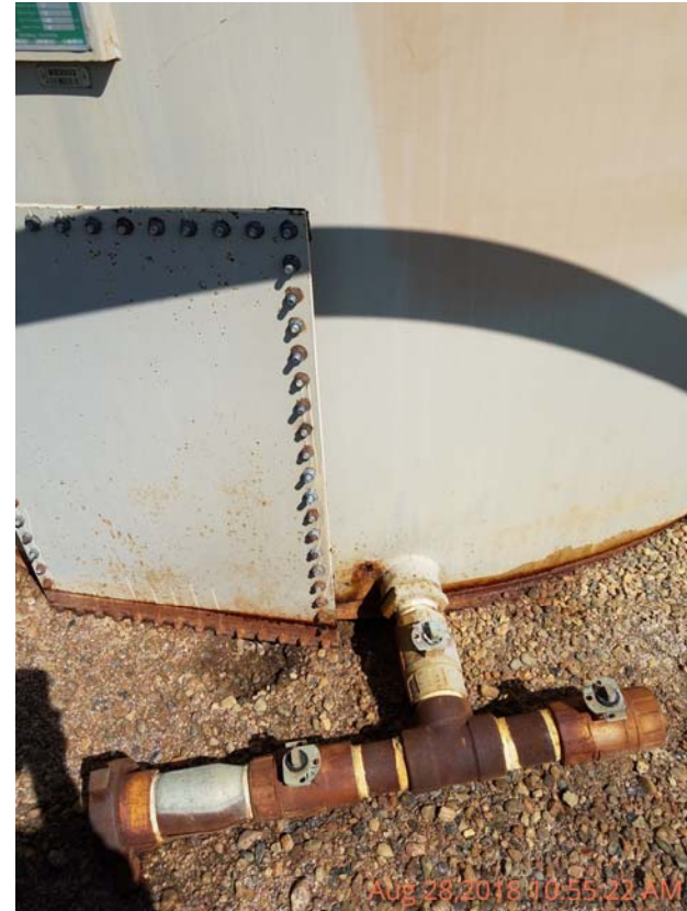
Photo 4 – Base of produced water tank. Corrosion hole visible.
