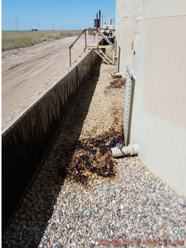
Photo 5 – Oil stained material within secondary containment. Southeast corner of tank battery looking west.
