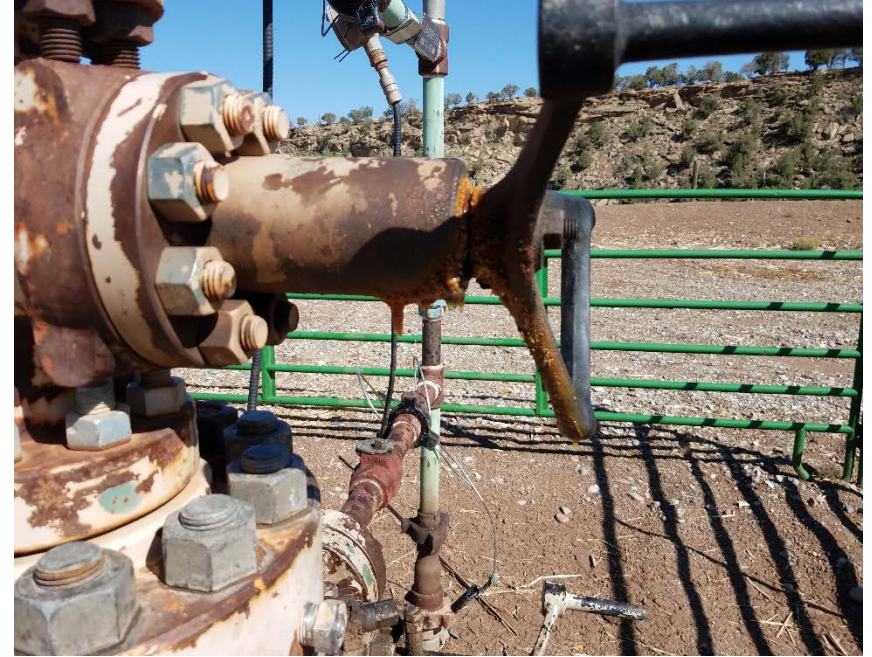
Location Photo #9, leaking bonnet on master valve
