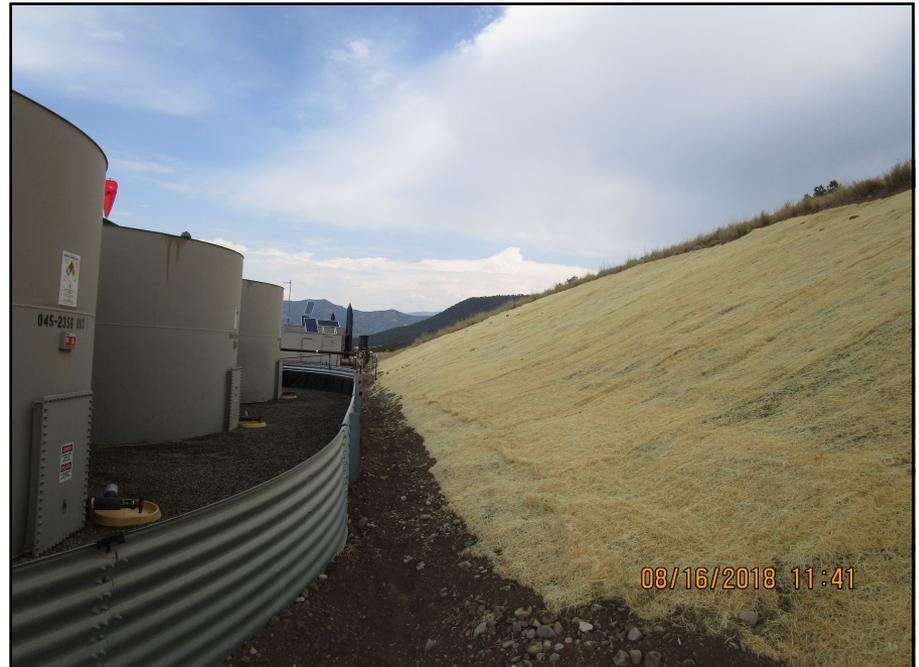
Sediment has been cleared from behind tank battery. The diversion ditch has been re-defined. Erosion control blankets have been installed on the cut slope.
