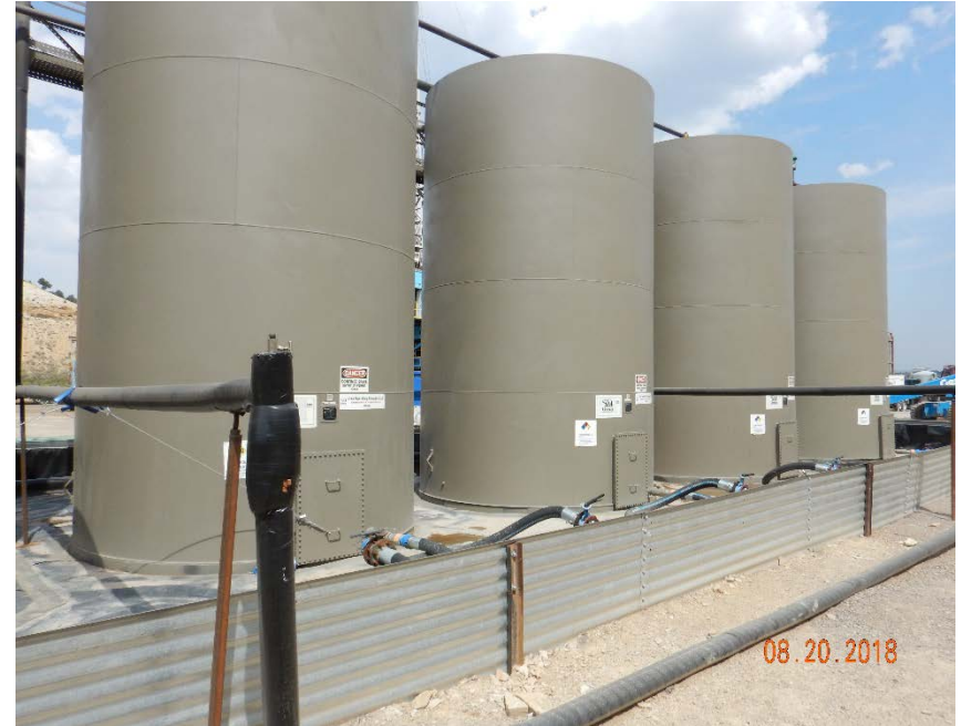
Photo #4 – Tank battery berm has been expanded to accommodate four (4) new tanks.
