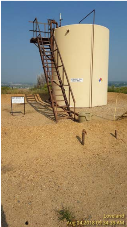
Photo 1 – Crude oil AST and tank battery sign.
