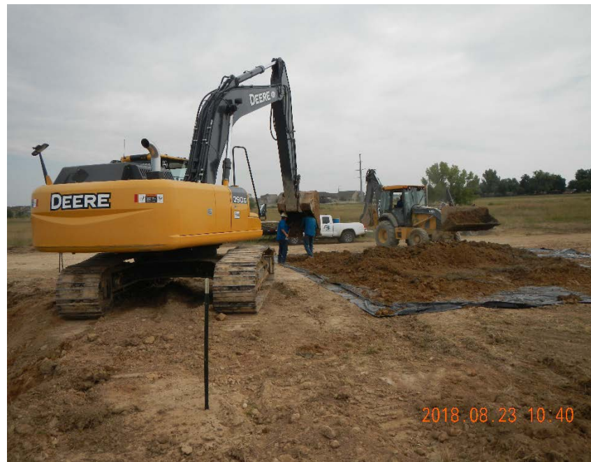
Photo 4. Spoil pile on liner.
