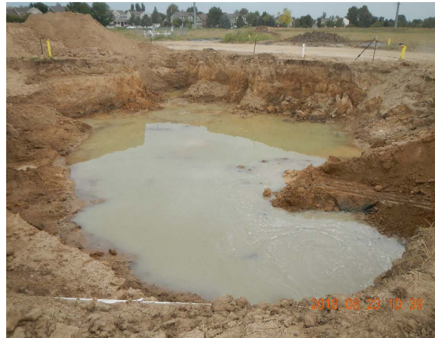
Photo 2. Ground water infiltrating open excavation.
