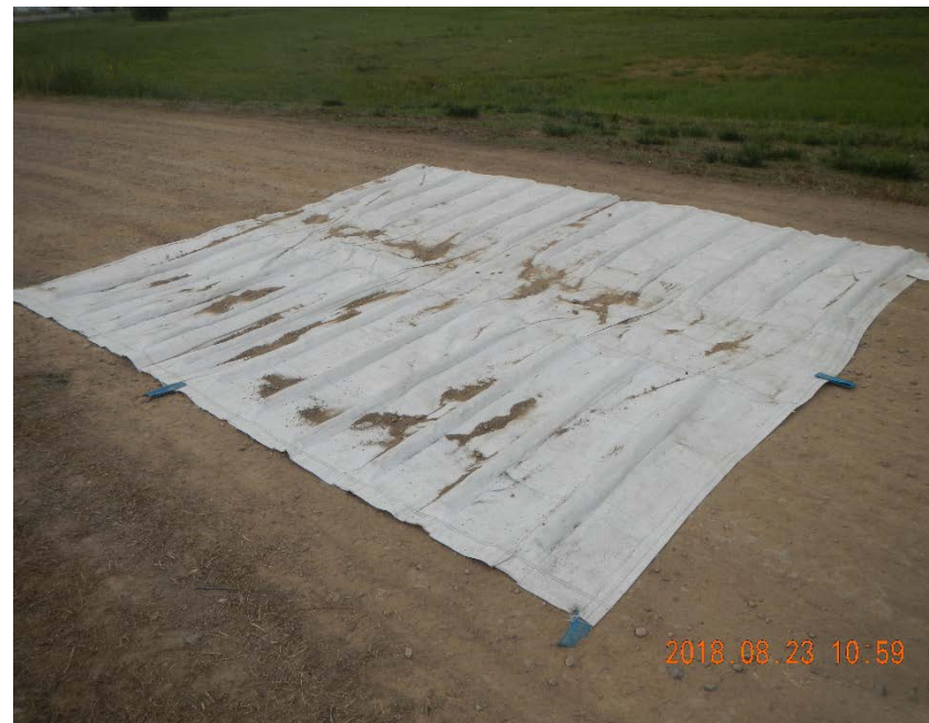
Photo 8. Vehicle tracking control pad.
