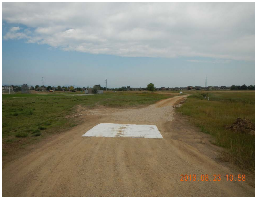
Photo 7. Vehicle tracking control pad.
