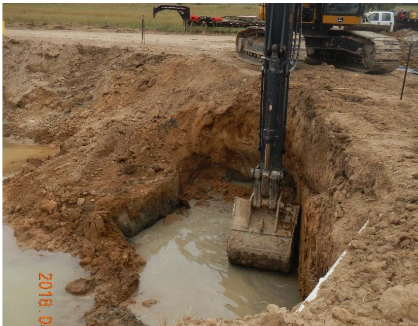
Photo 3. Excavating smear zone.
