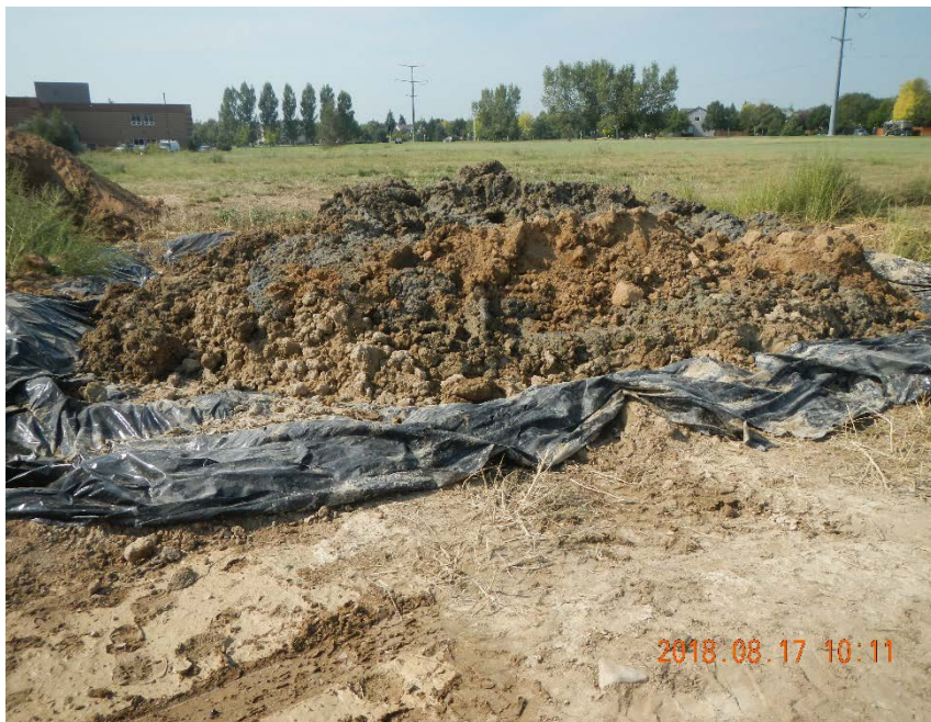
Impacted soil stock piled on a liner
