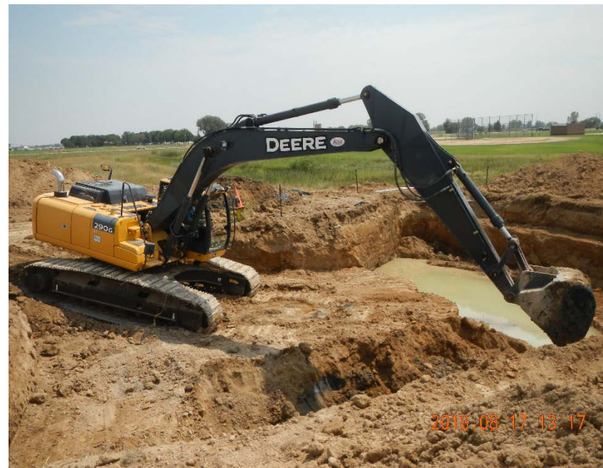
Tack excavator enlarging excavation
