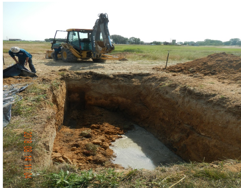
Ground water infiltrating the excavation
