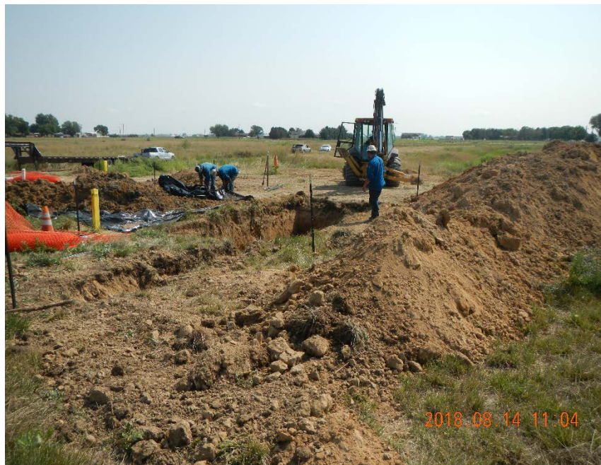
Excavation continuing with the backhoe
