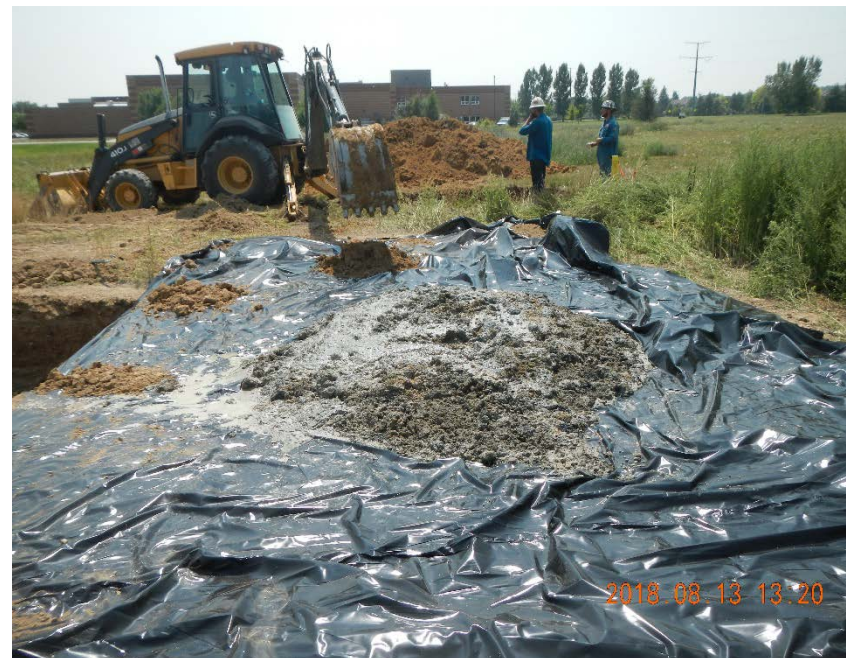
Impacted soil stock piled on liner
