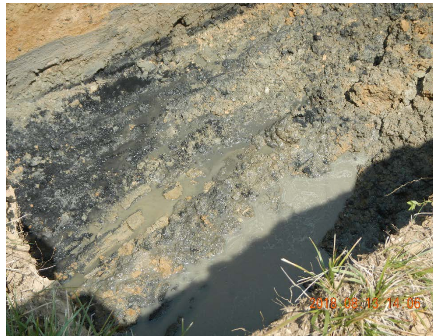
Ground water infiltrating the excavation
