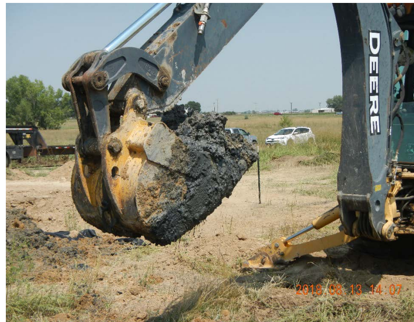
Close up of backhoe bucket lifting impacted soil from excavation
