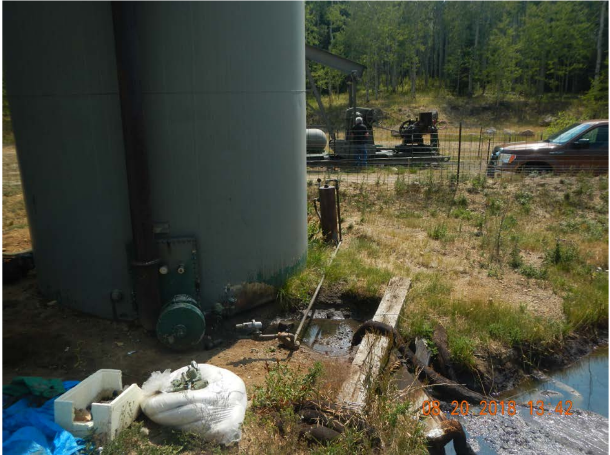
Looking south. Water from tank discharges to the ground to the pit.
