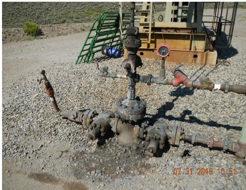
Stained equipment and wet soil surrounding well head.
