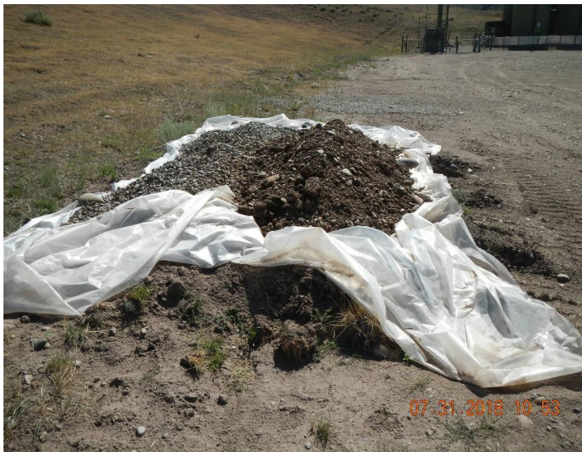
Stained soil temporarily stored on site in lined containment area.
