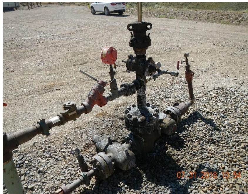
Federal 11-90-24 #1 well head with white residue and wet soil.
