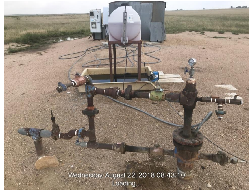
Photo#2 Corrective Action Stained Soil and Containment needs to be cleared out
