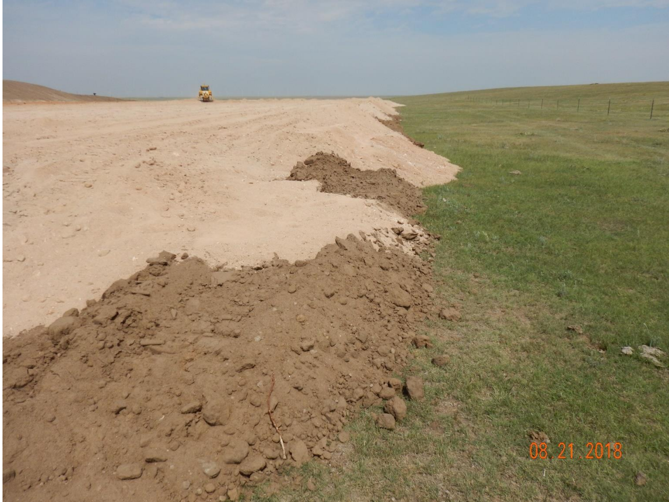
Photo 10: Photo taken from the southeast corner of the location, facing north. Photo shows insufficient perimeter stormwater and erosion controls have been installed.
