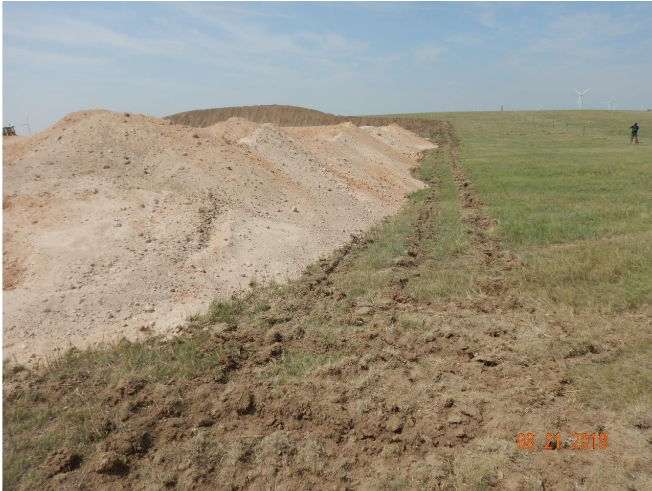
Photo 7: Photo taken from the southeast corner of the location, facing west. Photo shows surface roughening (ripping) installed along perimeter has filled with sediment and is not longer in proper functioning condition. BMP appears to be insufficient for the site and site's conditions.
