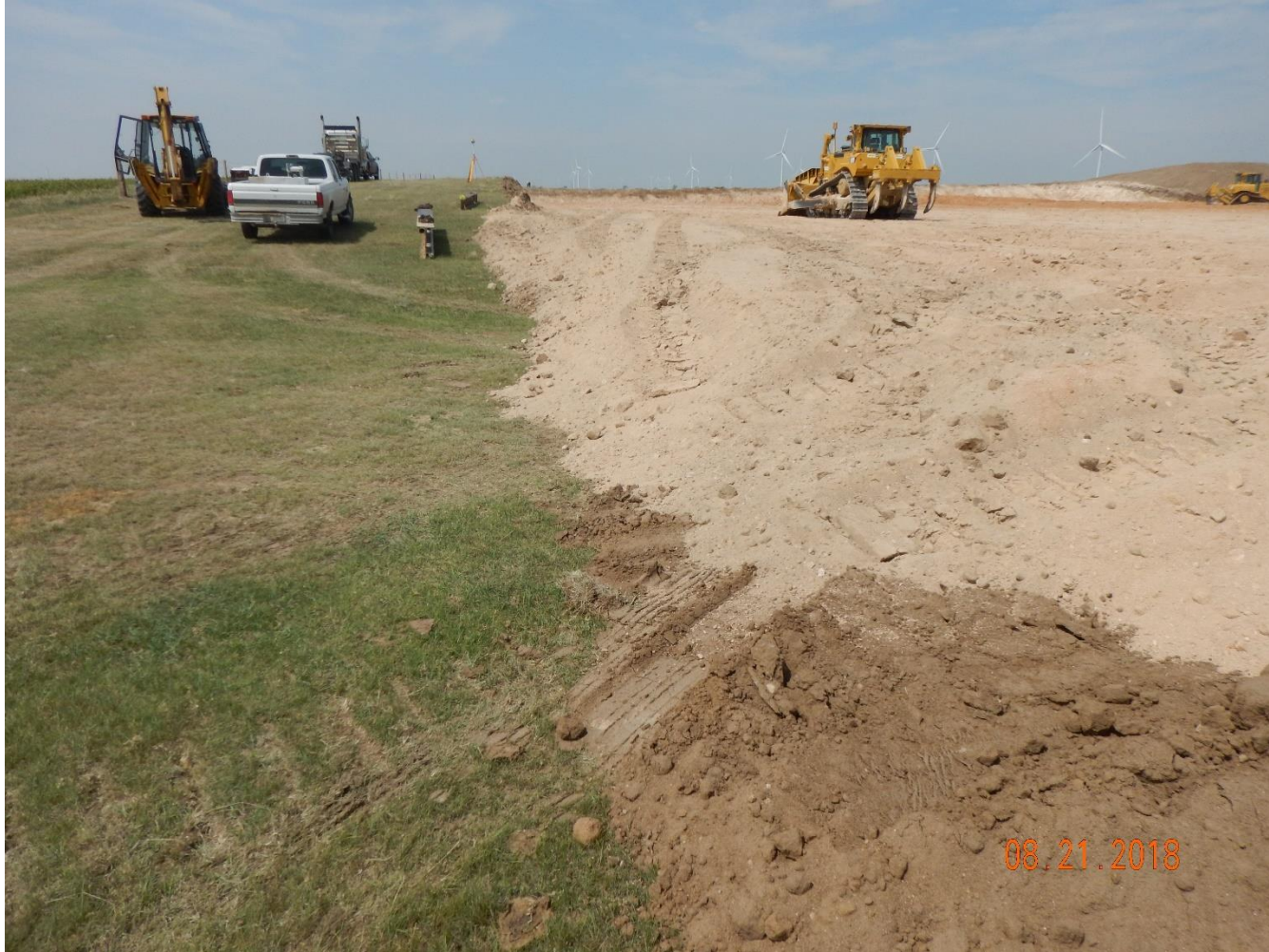
Photo 11: Photo taken from the southeast corner of the location, facing west. Photo shows insufficient perimeter stormwater and erosion controls have been installed.
