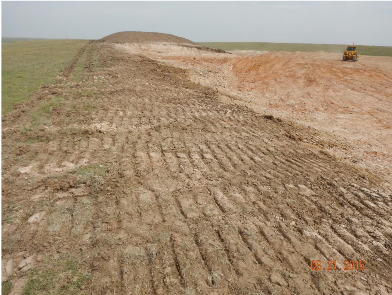
Photo 2: Photo taken from the southwest corner of the location, facing north. Photo shows construction in process. Photo also shows surface roughening (ripping) appears to have been installed on the western perimeter of the location. Surface roughening is a temporary BMP that should be used in conjunction with other BMPs and should not be used / replaced once pad construction and stabilization has completed
