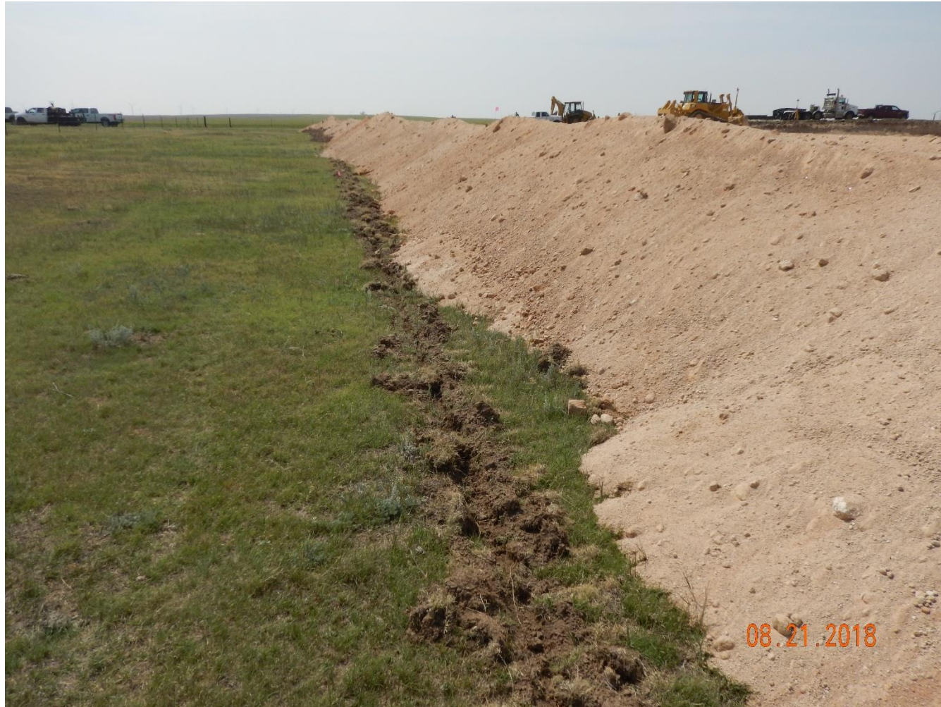
Photo 9: Photo taken from the east end of the location, facing south. Photo shows surface roughening (ripping) installed along perimeter has filled with sediment and is not longer in proper functioning condition. BMP appears to be insufficient for the site and site's conditions.
