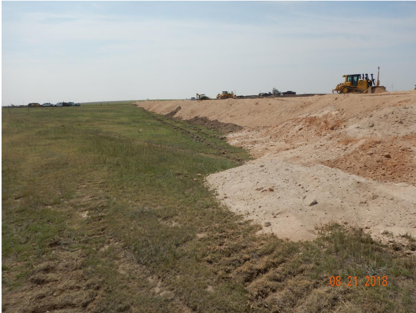
Photo 8: Photo taken from the southeast corner of the location, facing south. Photo shows surface roughening (ripping) installed along perimeter has filled with sediment and is not longer in proper functioning condition. BMP appears to be insufficient for the site and site's conditions.
