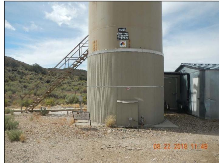
**Photo 2. Tanks with no berm.**
