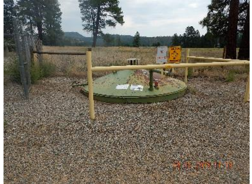
Photo 8: Tank with no berms.
