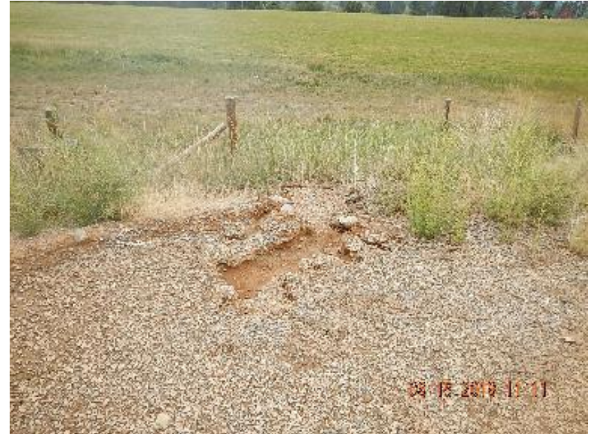
Photo 10: Erosion channeling on fill slope.
