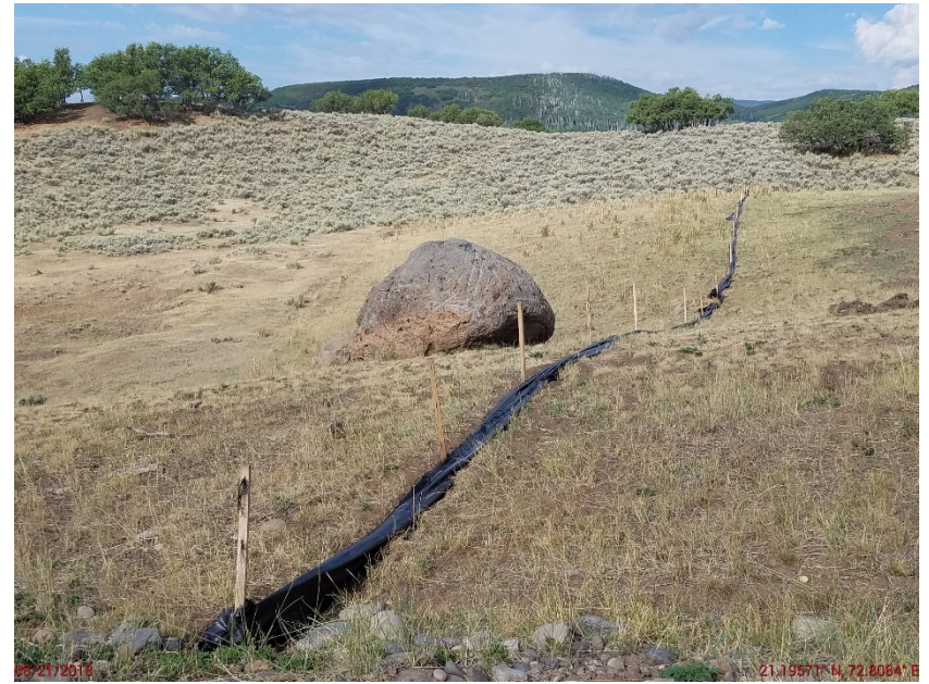
Photo 2. Silt fence in disrepair.
