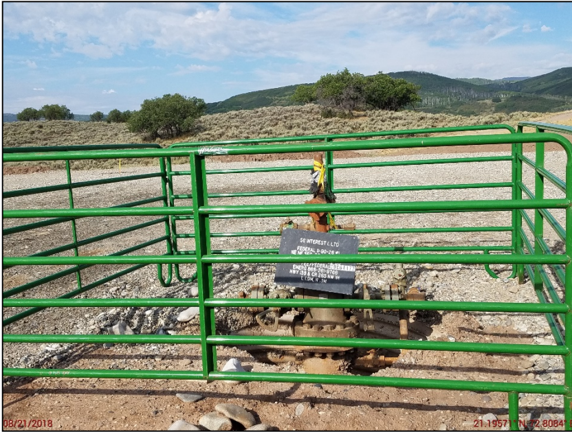
Photo 1. Wellhead. All production equipment has been disconnected.
