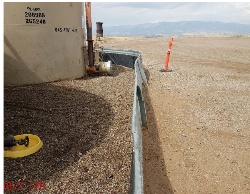
Location Photo #4, Containment damage
